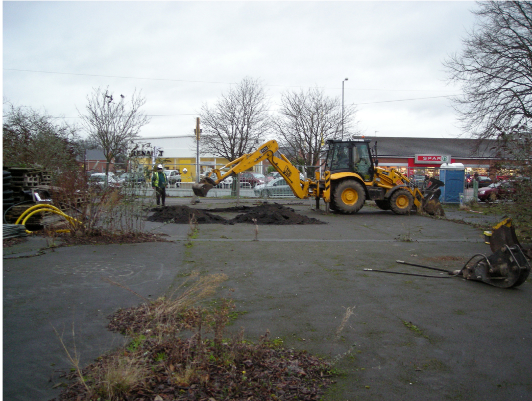
Plate 1. Machining Trench 1 looking north
