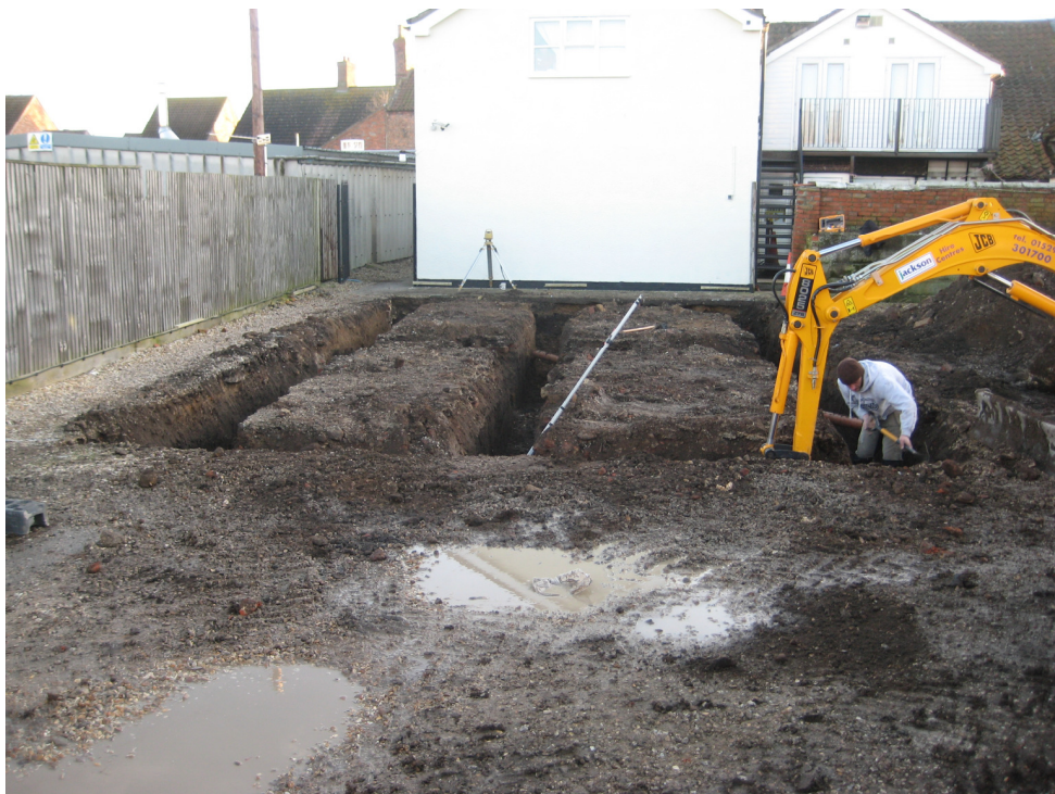
Plate 5. Completed footings looking southeast
