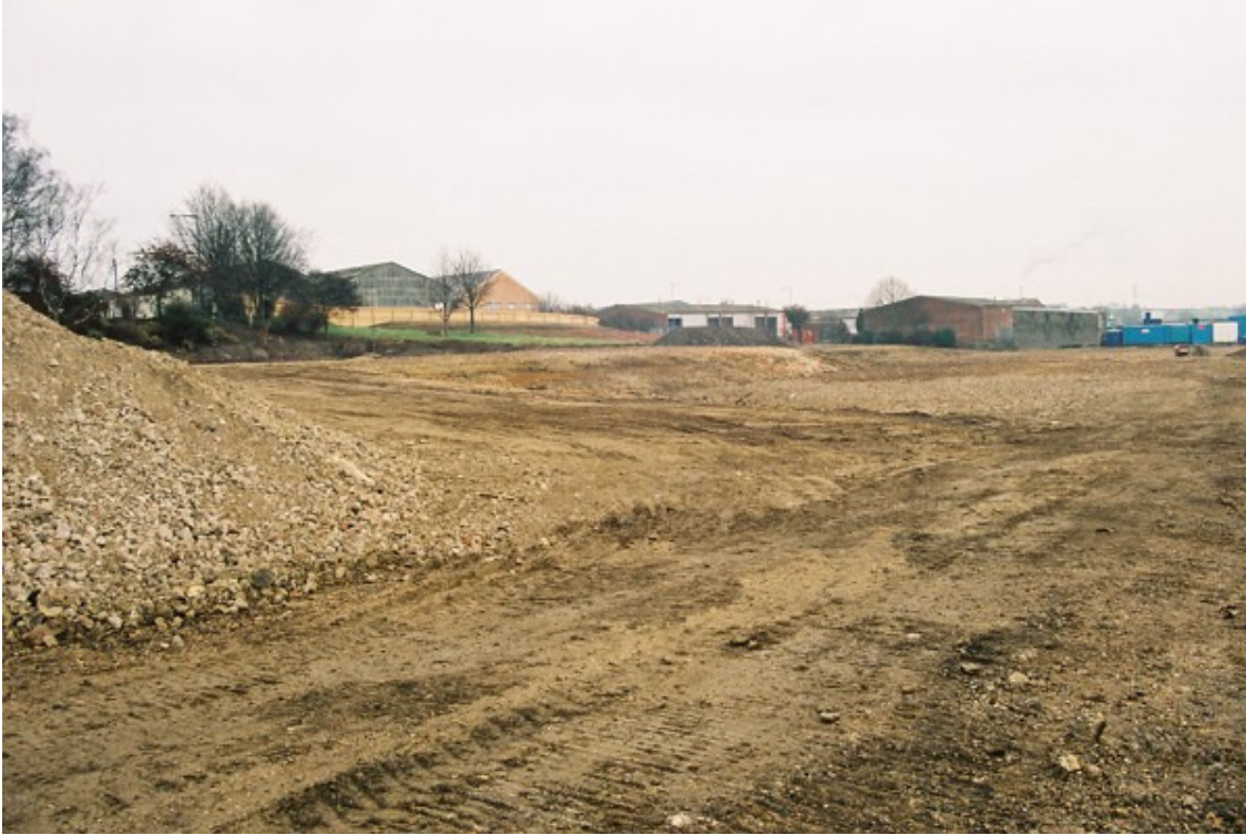
Plate 1 – General view of site
