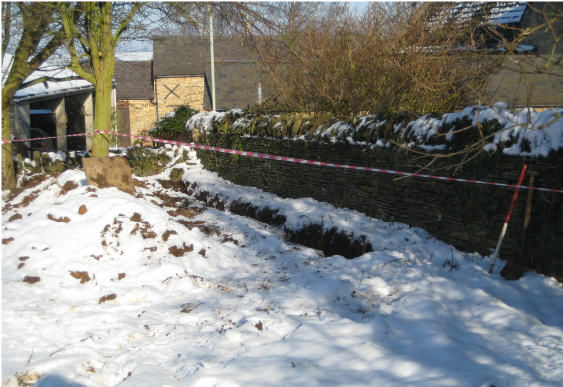
Plate 2 – General shot of trench for root barrier
