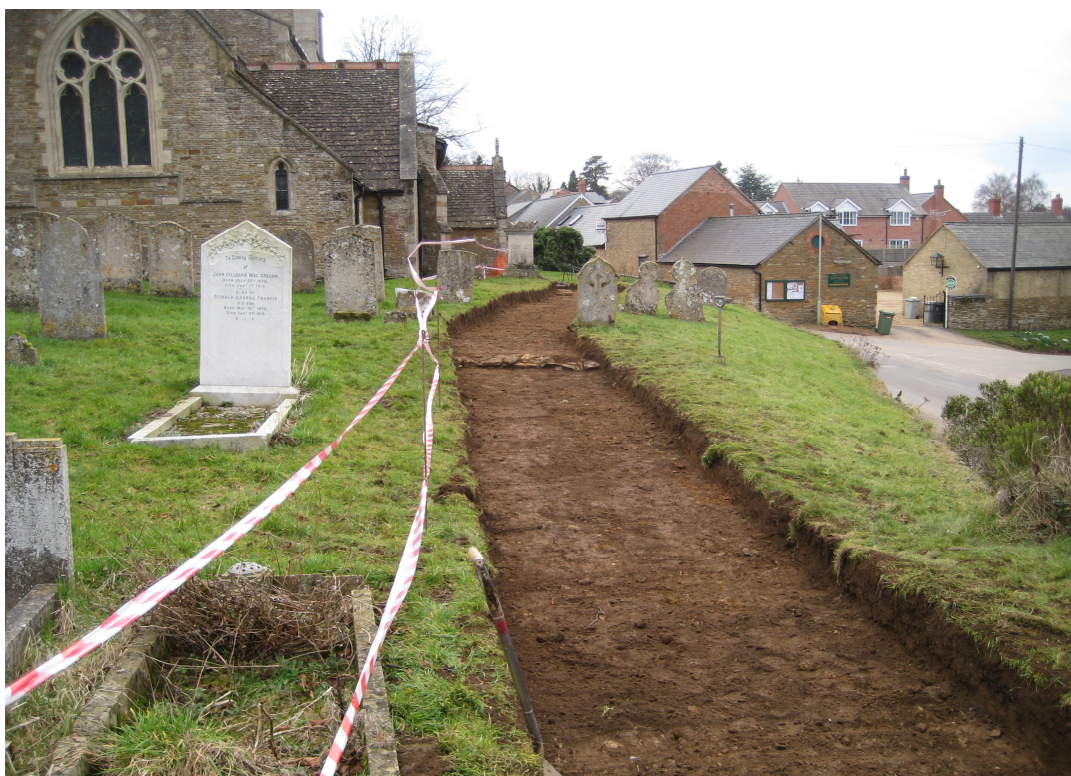
Plate 7 – General view of stripped footpath
