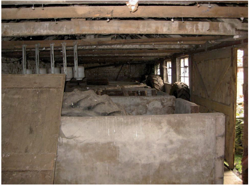
Plate 29 Interior of eastern range of animal accommodation showing concrete animal pens, looking south
