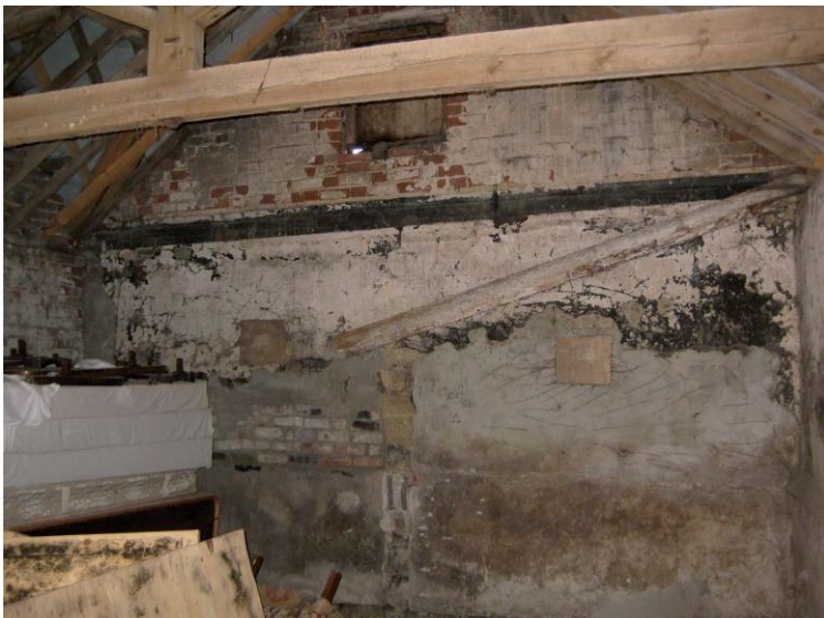
Plate 10 Western animal accommodation range internal, west wall partly of brick and unfired clay block, with slate attached to wall, looking southwest
