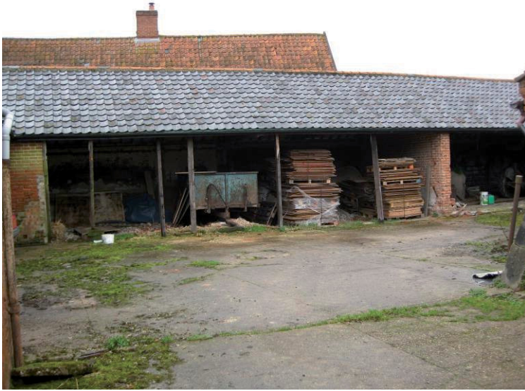
Plate 9 Western animal accommodation range, looking west
