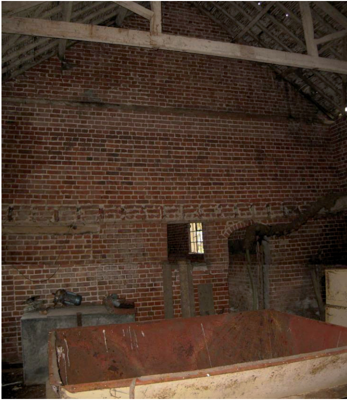
Plate 20 Interior of main barn, west gable end, showing change in brick coursing, holes for joists to upper floor and blocked doorway, looking west
