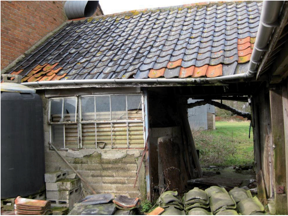
Plate 27 Southern wall of northeastern animal accommodation, looking north
