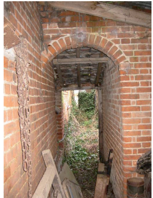
Plate 36 Covered passageway at western edge of east range, looking north
