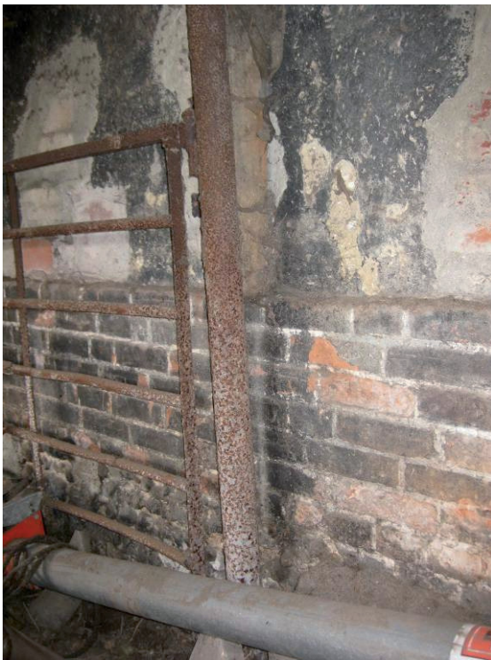
Plate 13 Northern room of western animal accommodation range, detail of west wall construction including flint cobble, brick and unfired clay block, looking southwest
