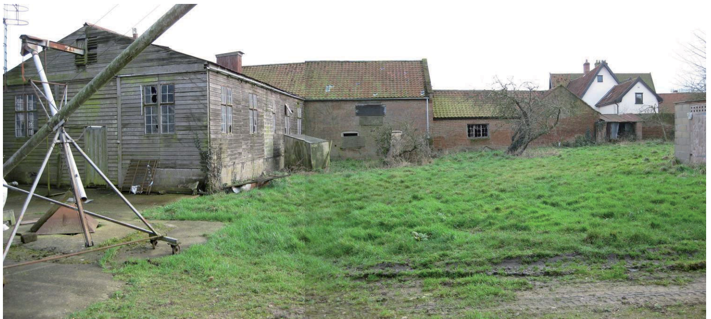
Plate 38 General view of buildings from north, northern walls of animal accommodation and main barn and timber shed, looking south
