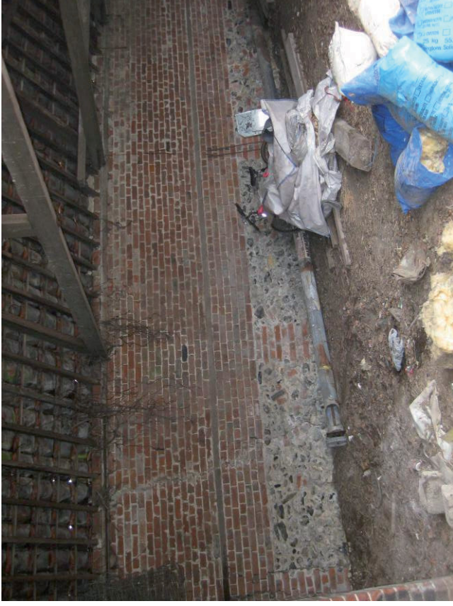
Plate 3 Western wall of cart shed, interior, flint cobble and brick walling, looking west
