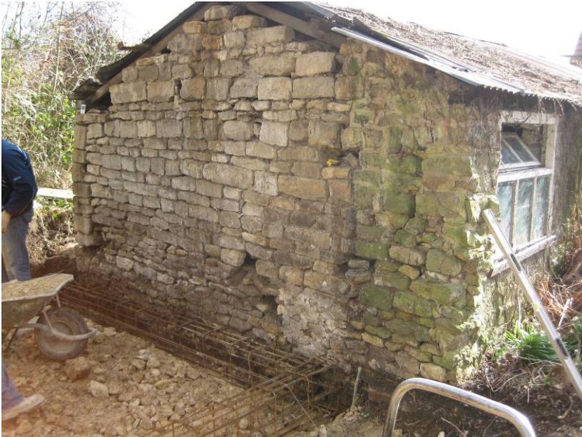
Plate 6 Northern wall of recorded building, looking southeast
