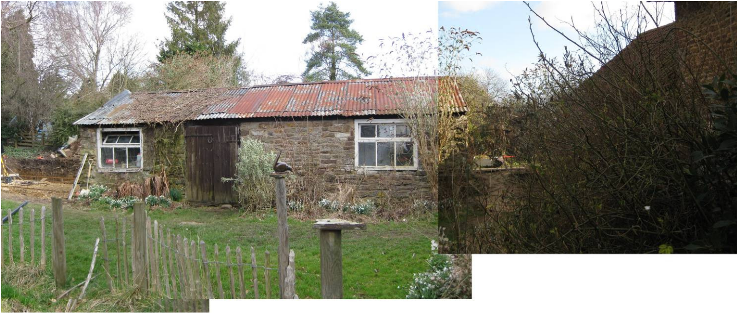
Plate 3 General view including western wall of recorded building, looking east
