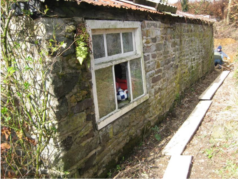
Plate 5 General view including eastern wall of recorded building, looking northwest
