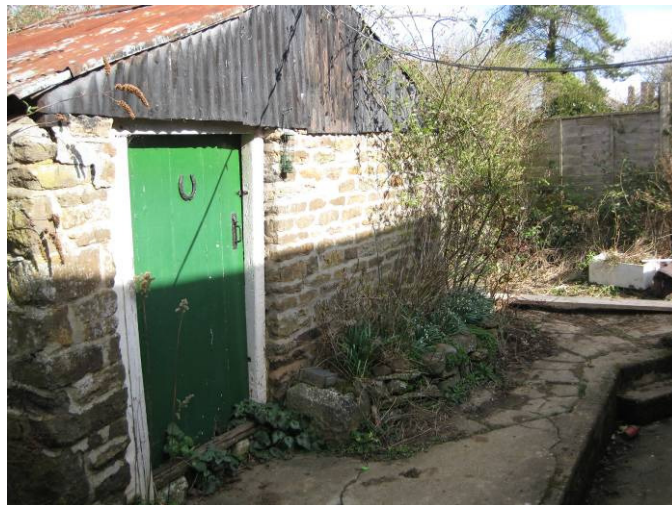
Plate 2 Southern wall of recorded building, looking northeast
