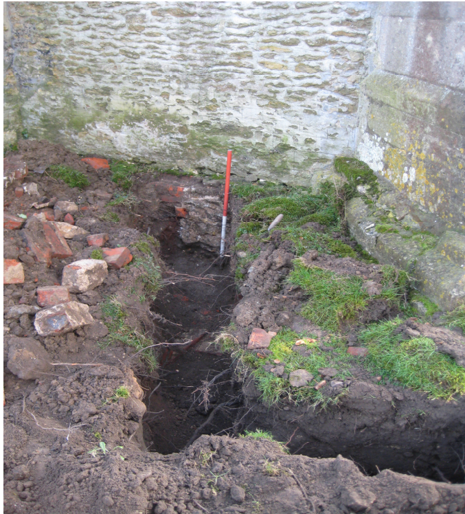
Plate 5 – Remains of brick structure (026) in base of pipe trench
