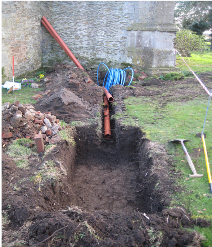
Plate 7 – Soakaway to the north of church tower
