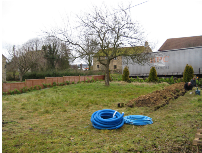
Plate 1 – View of the service trench, looking southeast
