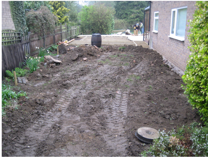
Plate 1 – General view across the development area, looking northwest
