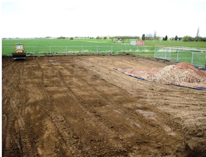
Plate 2 – The stripped area for the new compound, looking north
