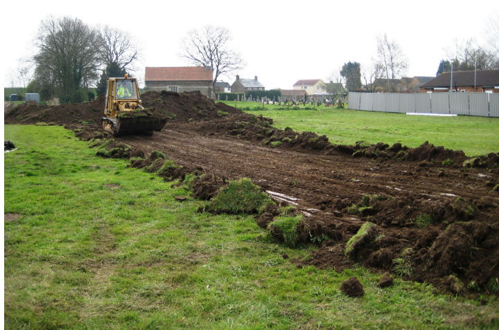
Plate 1 – Initial stripping of the access road, looking south
