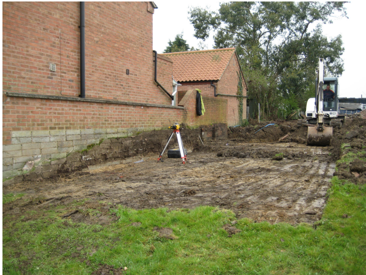
Plate 1 – View across the development area, looking southwest
