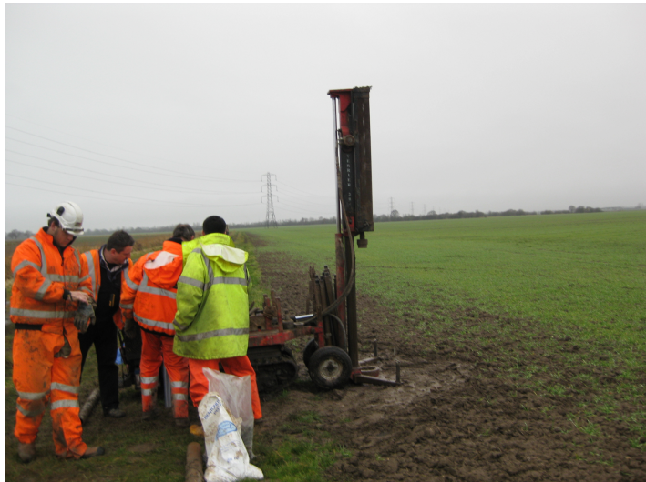
Plate 2 – Borehole rig at Borehole 2
