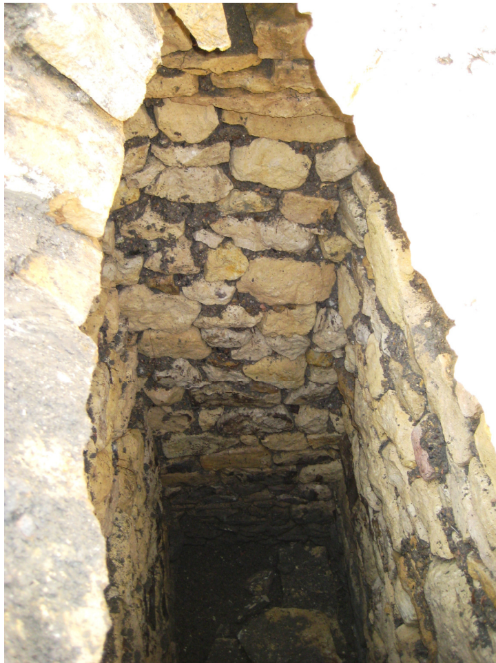
Plate 6 – Interior view of cistern (017), looking north
