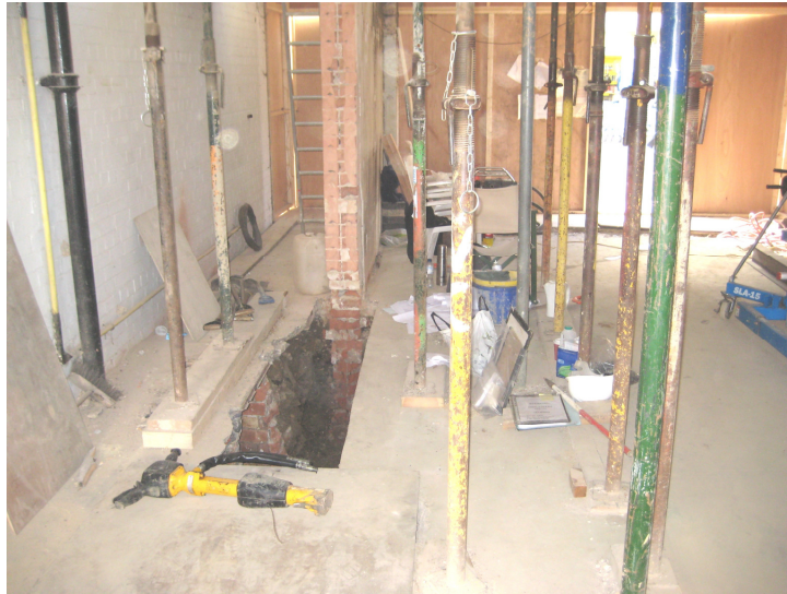
Plate 7 – View showing groundworks within the shop, looking south
