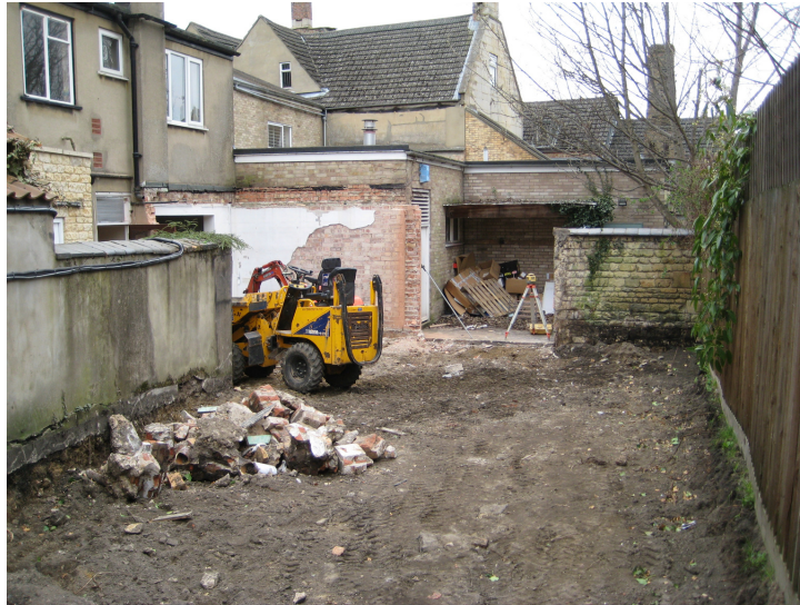
Plate 1 – View across the rear part of the development area, looking west
