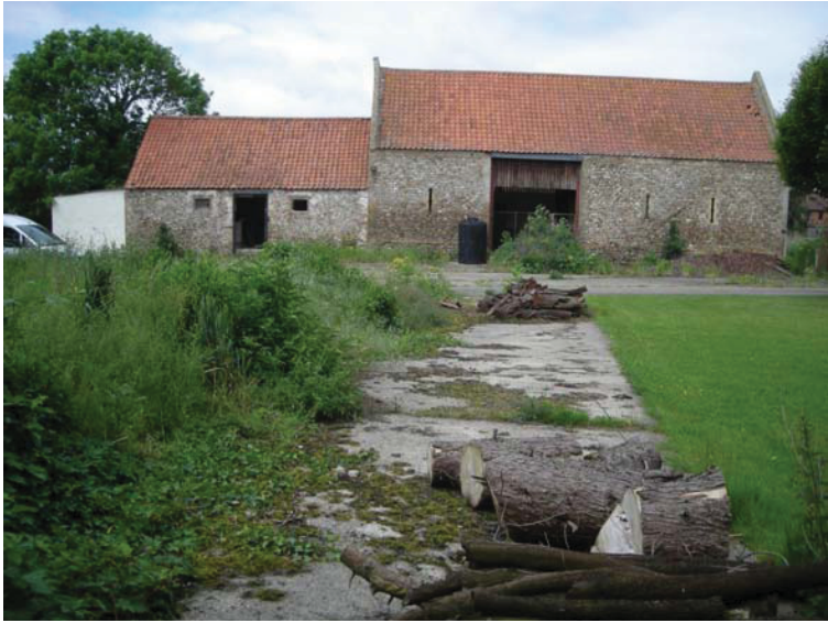
Plate 2 General view of the recorded buildings, looking west
