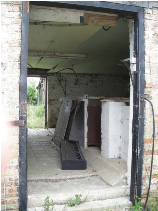
Plate 19 Corridor through southerly building, looking west
