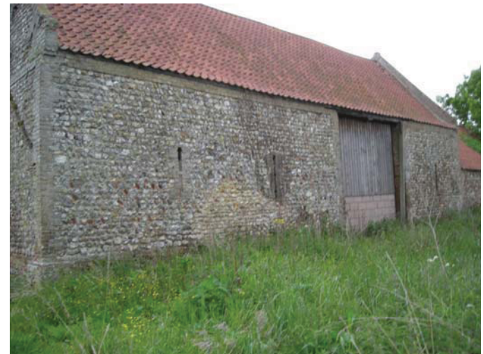
Plate 12 West elevation of main barn, showing infilled area, looking southeast
