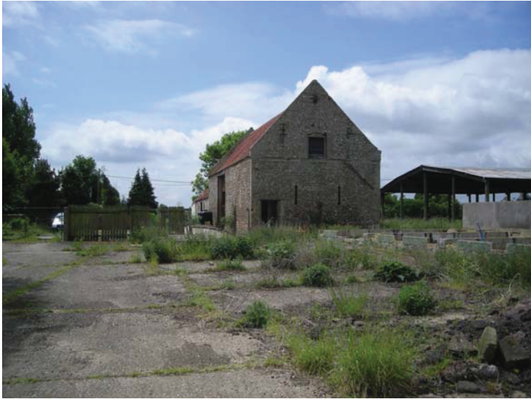
Plate 3 General view of the recorded buildings, looking south
