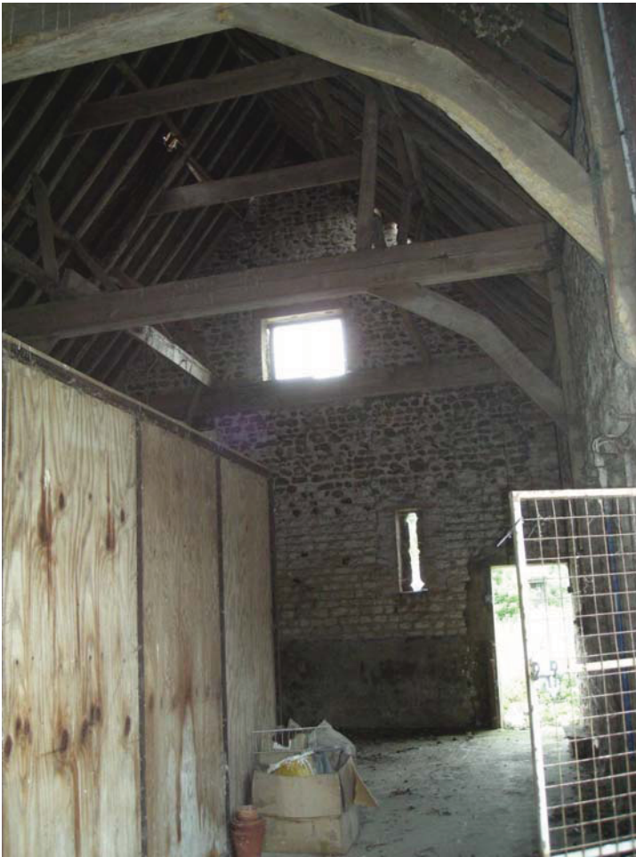
Plate 13 Interior of main barn, looking north
