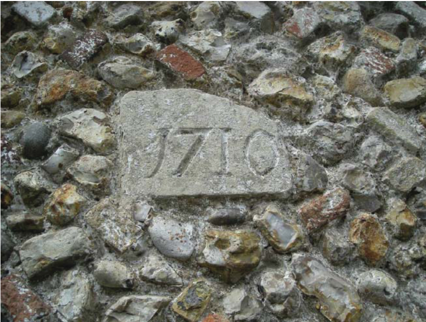
Plate 9 Detail of east elevation of southerly building showing re-used date stone in walling, looking west
