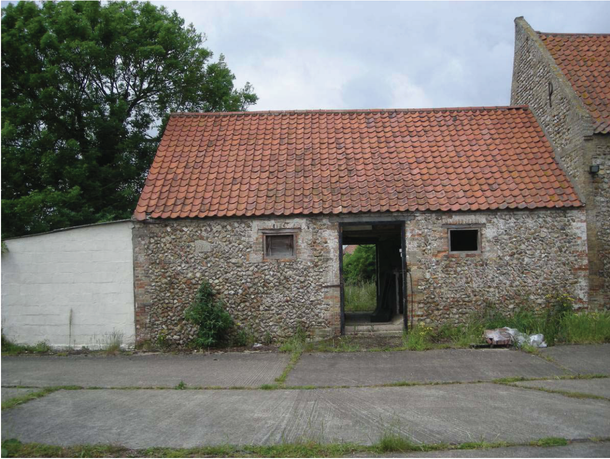
Plate 8 East elevation of southerly building, looking west
