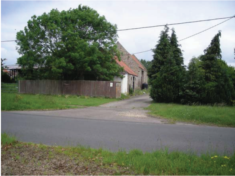
Plate 1 General view of the recorded buildings from Low Road, looking north
