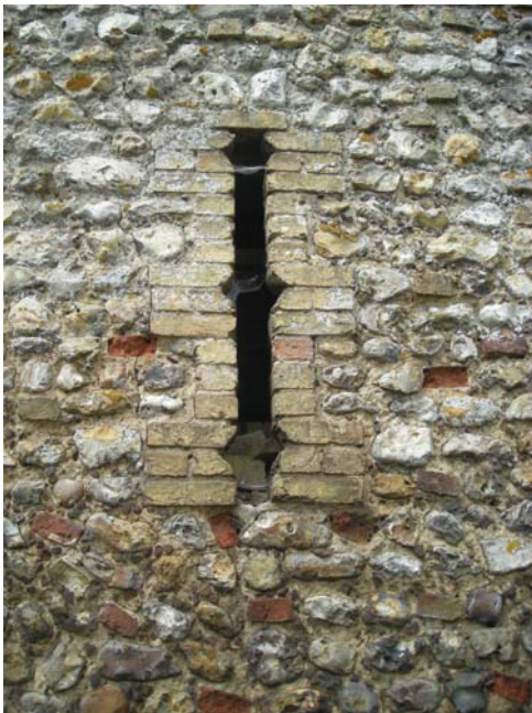
Plate 6 Detail of breather slit, main barn, looking west
