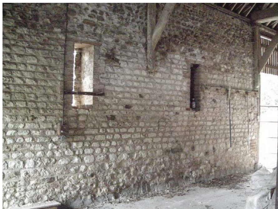
Plate 15 Interior of main barn showing chalk and flint construction, looking southeast
