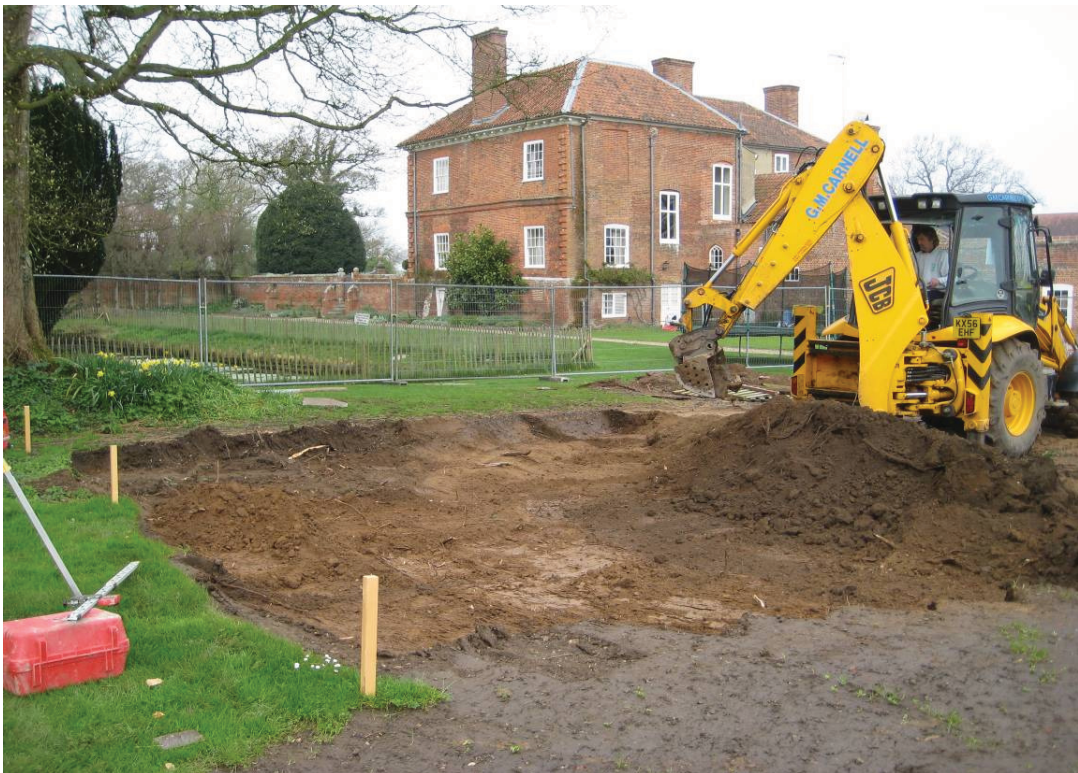
Plate 2 - Stripping of earth in south-eastern area of site
