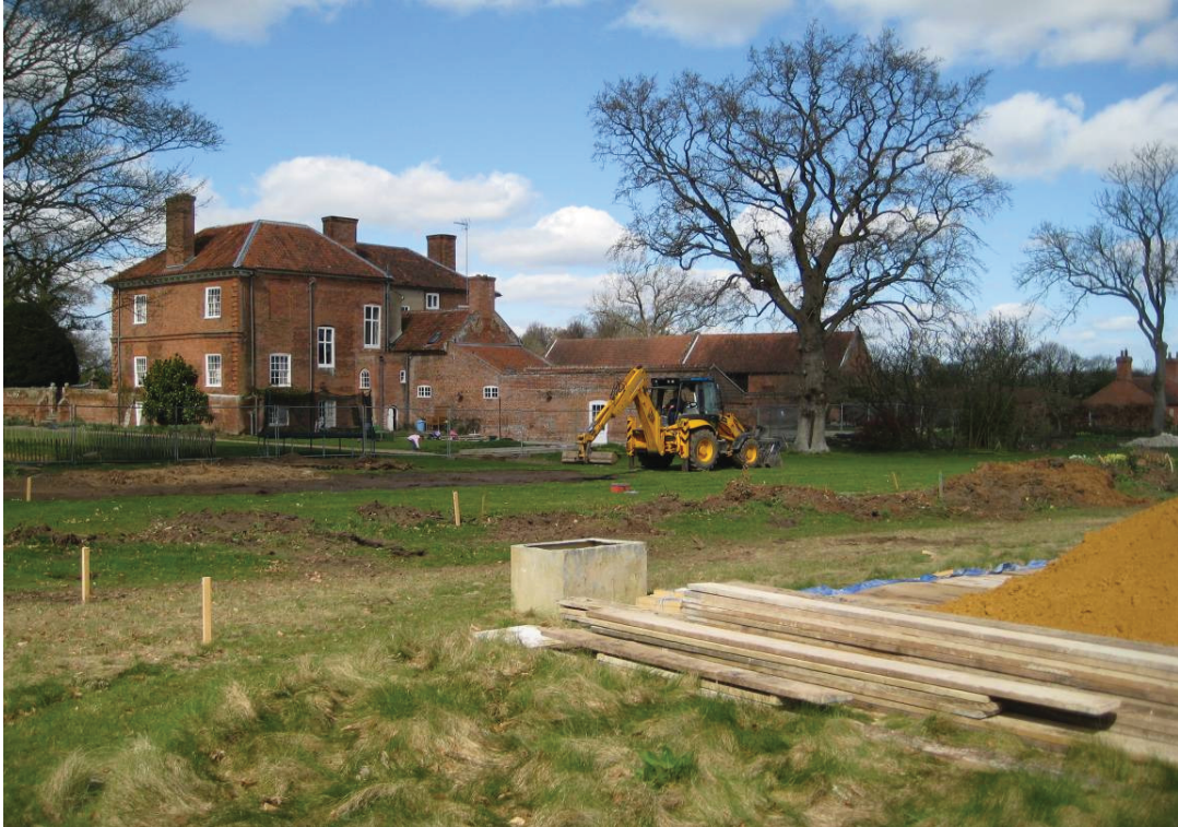
Plate 1 – General view of site
