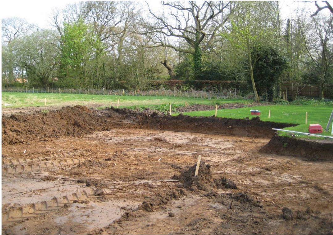
Plate 3 – General view of stripping in southern area of site
