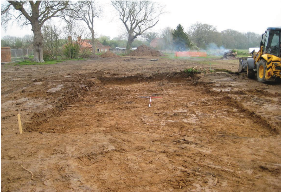
Plate 5 – Excavation of pool area
