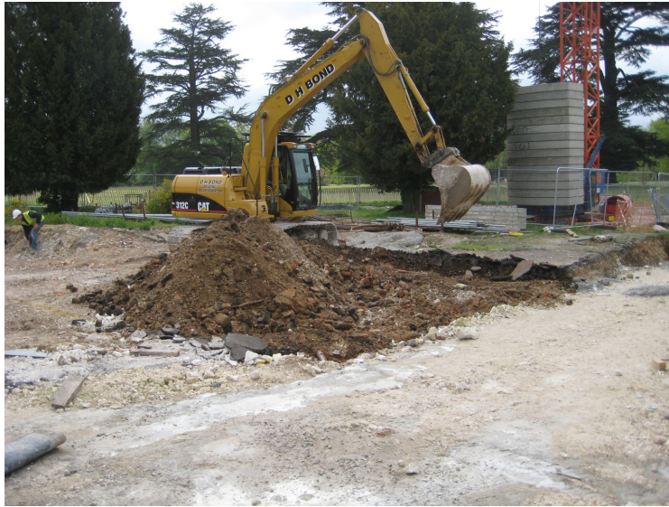
Plate 1. Starting the strip for the new guest house looking southeast
