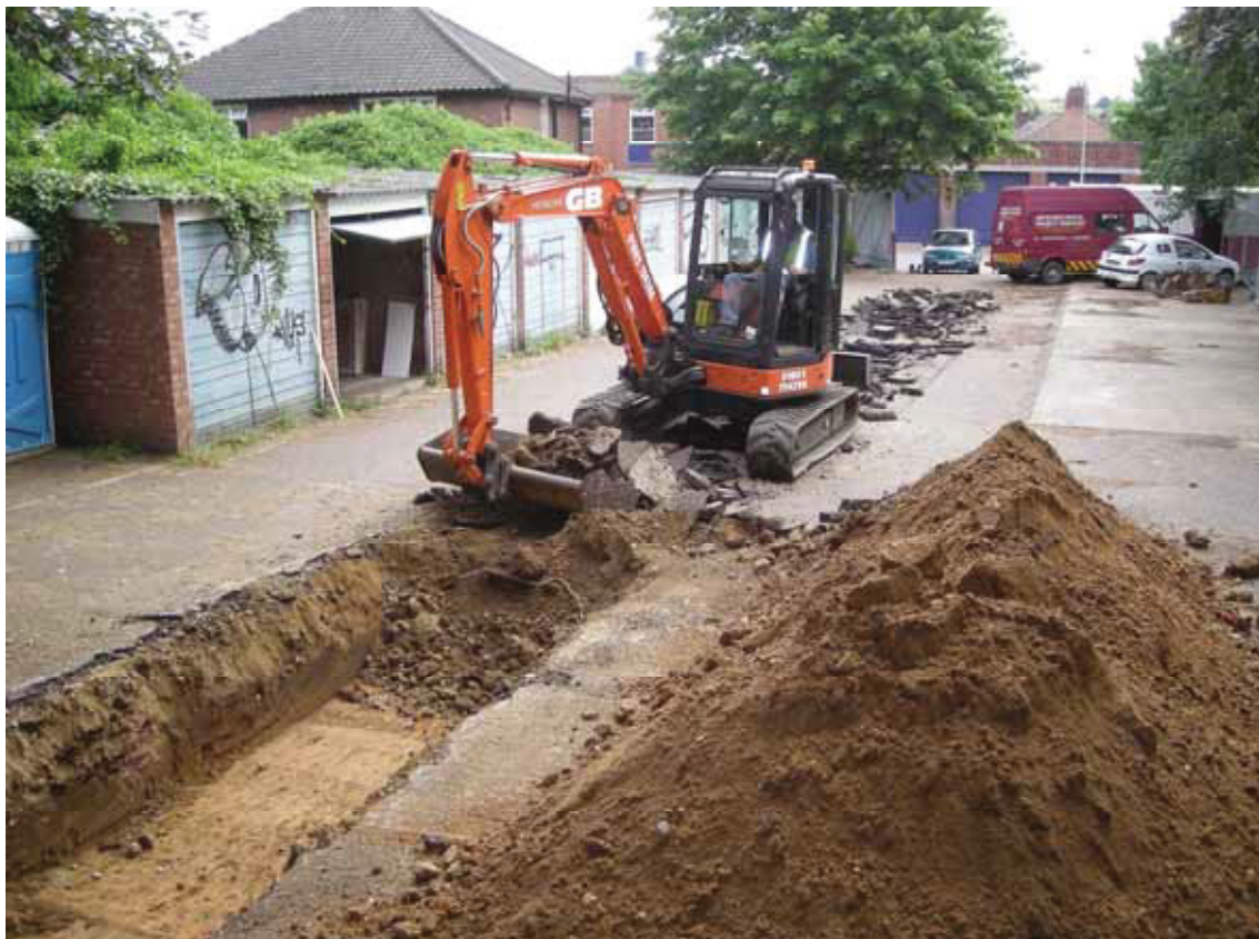
Plate 2. Machining Trench 3 looking east
