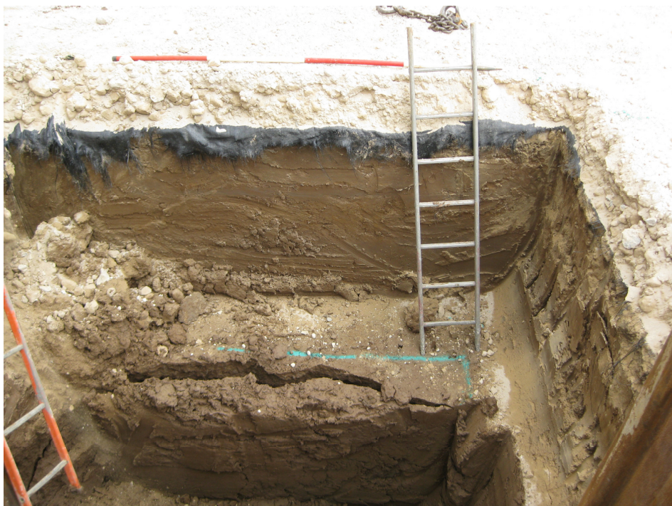
Plate 4. Hole for water tank, Section 8 looking north
