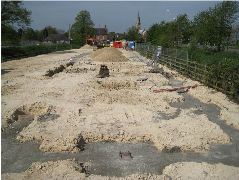
Plate 1. General view of site, with footings almost completed, looking west
