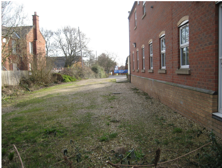
Plate 2. Pre excavation view of route of pipe trench looking east
