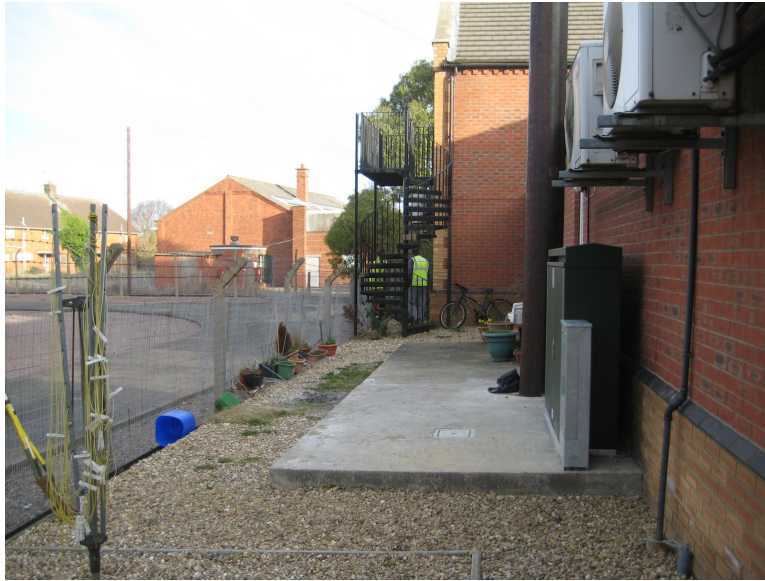
Plate 1. Pre excavation view of route of pipe trench to rear of building looking north
