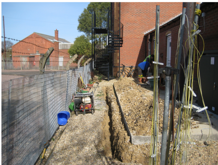
Plate 3. Start of pipe trench to rear of building looking north
