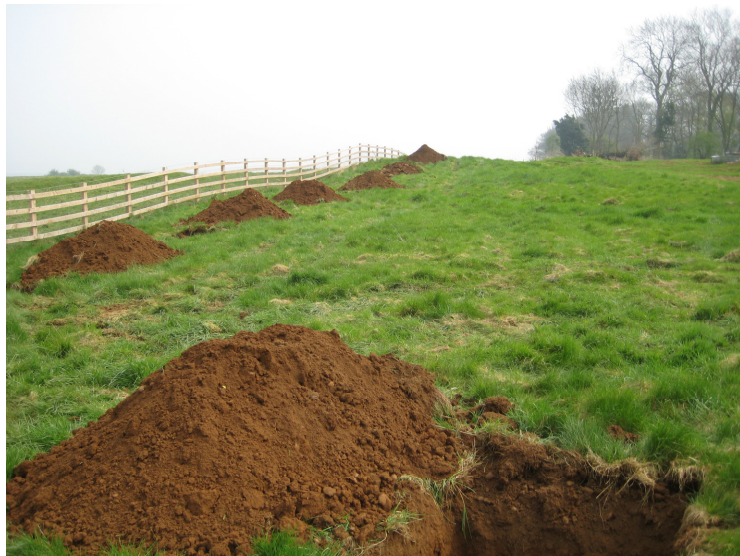
Plate 2 – General view of the eastern area of works, looking east
