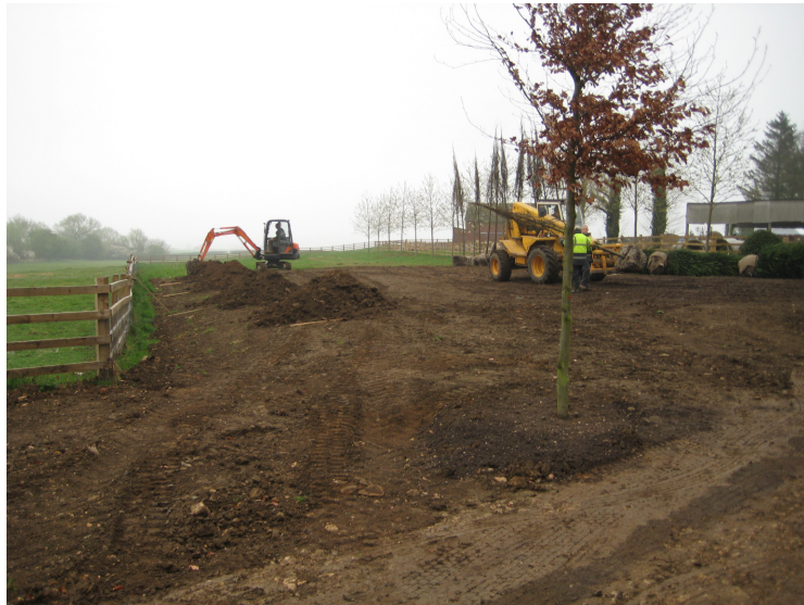
Plate 1 – General view of the southern area of works, looking north
