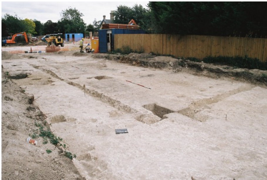
Plate 6 Southeast facing view western area of site after excavation of Buildings 1, 2 and 3
