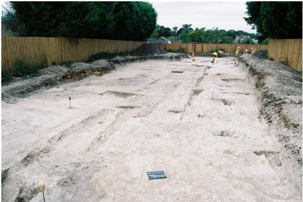
Plate 8 West facing view western area of site after excavation of Buildings 2, 3, 5 and 6
