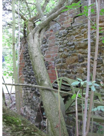
Plate 43 West wall of store 1, looking northeast
