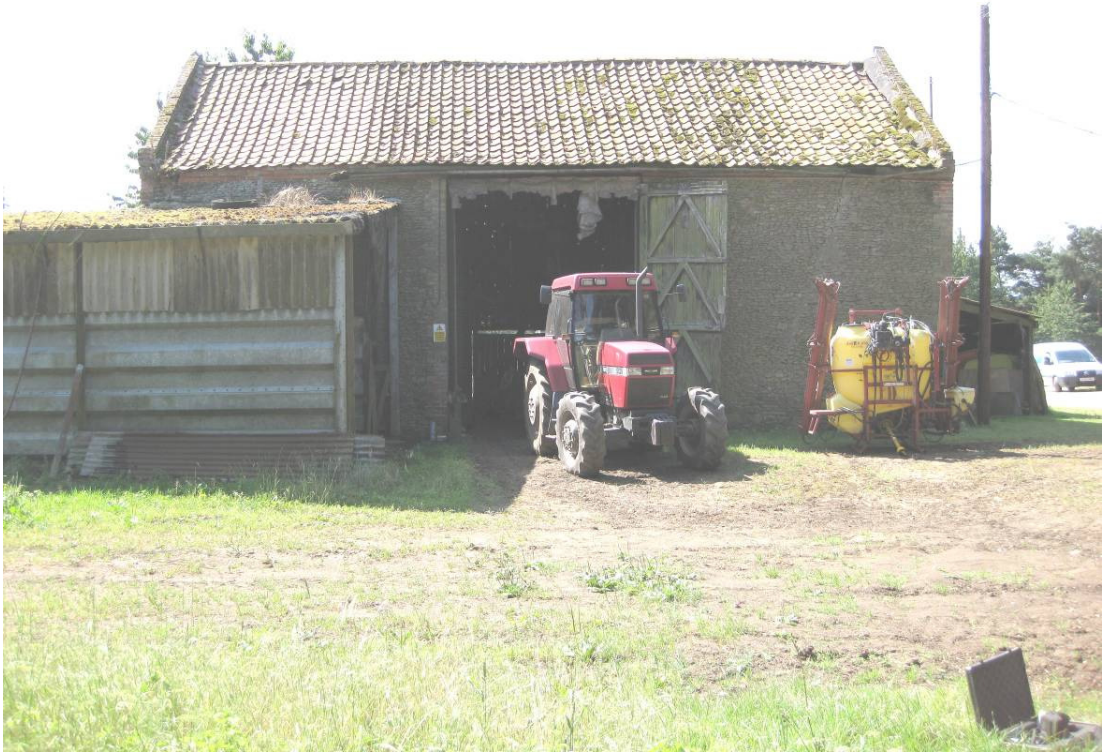
Plate 4 Northern wall of main barn showing raised gable and large opening. Tractor store 1 at left, lean-to store 4 at far right of barn, looking south.
