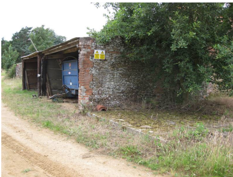
Plate 32 Stores 2 & 3, looking northwest
