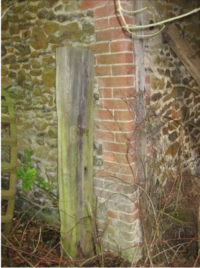
Plate 42 Detail of quoins at northwestern corner of cartshed at join with store 1. Some possible diagonal skintling marks in these bricks although these do not show in this photograph, looking northeast.
