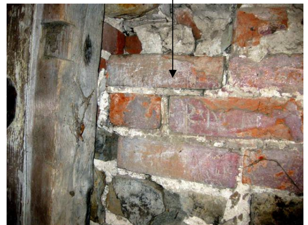
Plate 20 Detail of quoin inside barn porch, at west side of wooden doors showing vertical scratches on brick, possibly relating to number of sacks loaded or similar. Also further graffiti including initials, looking southwest.
