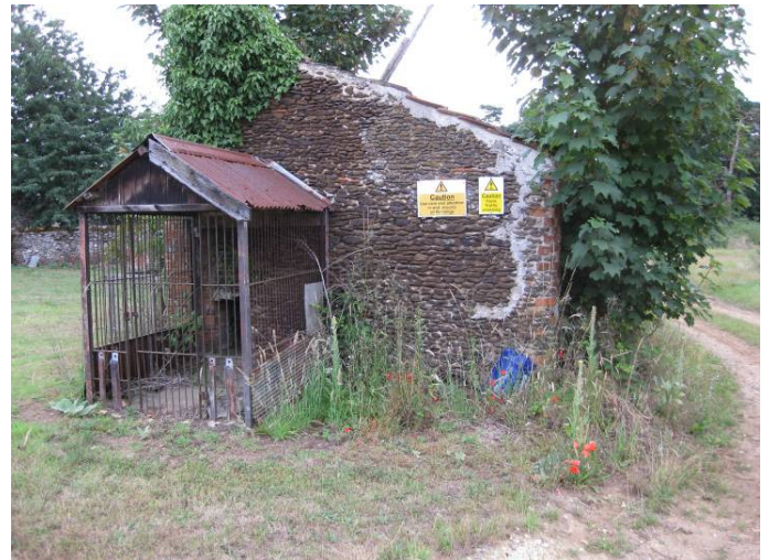
Plate 46 West end of southern building, looking east.
