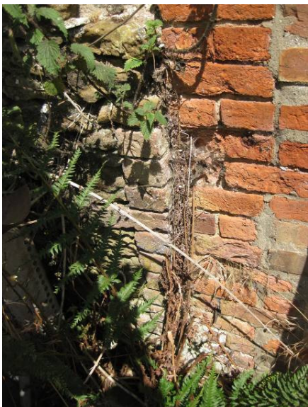
Plate 9 Detail of join between stable 1 and tack room, looking north.
