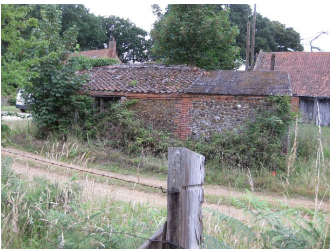
Plate 45 South wall of southern building, looking north.
