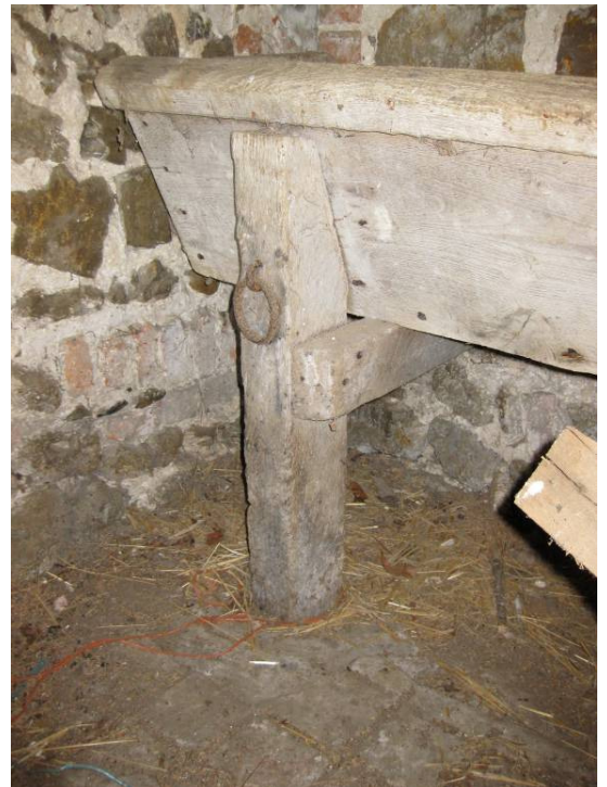
Plate 24 Interior of stable/loose box 2, detail showing wooden manger, possibly original to building and flag/tile flooring, looking northwest.
