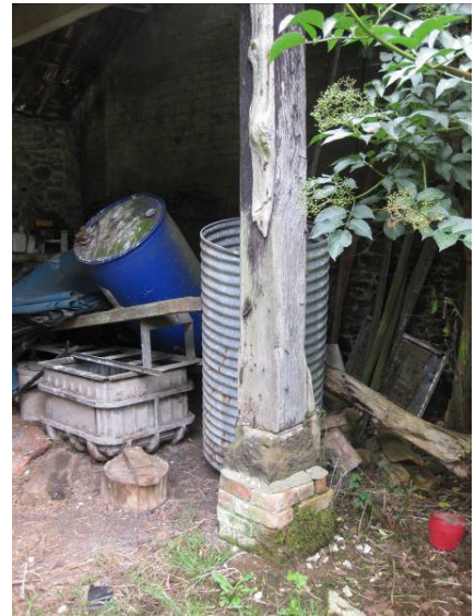
Plate 41 Detail of cartshed frontage, timber post over brick and stone plinth, looking southeast.
