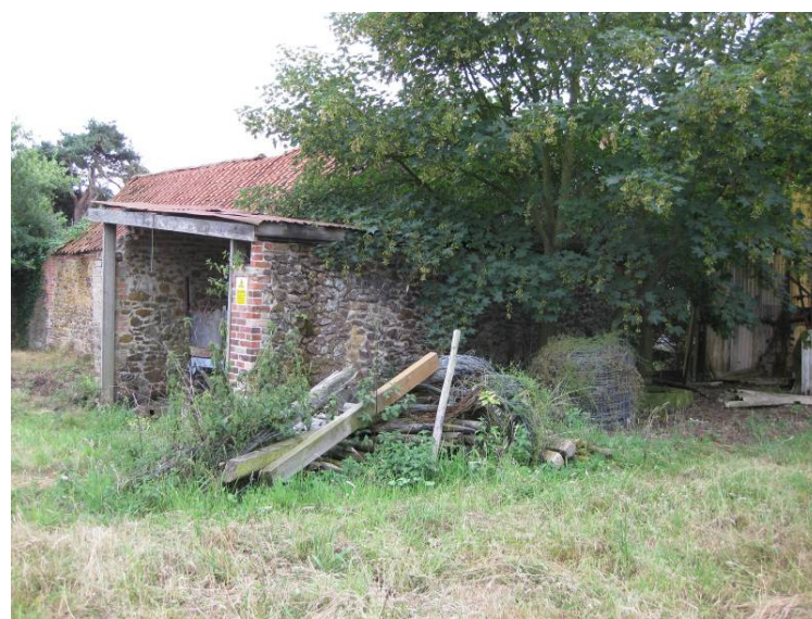
Plate 34 Store 1, cart shed to rear, looking southwest
