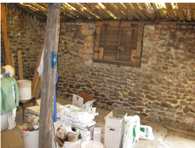
Plate 29 Interior of chemical store showing east wall, looking northeast
