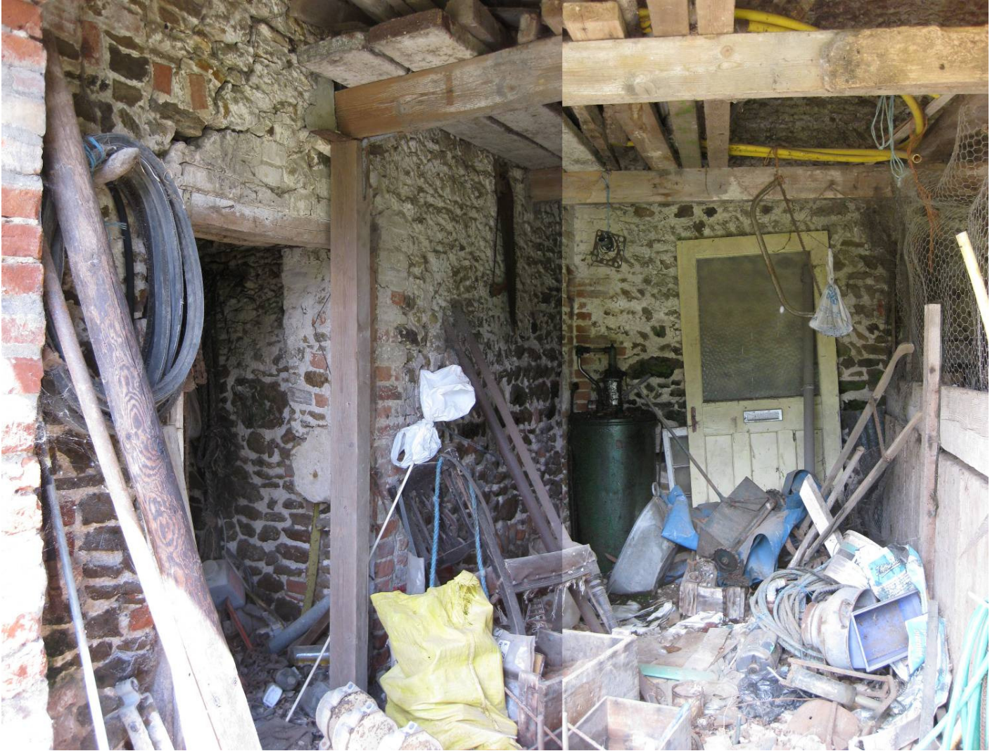
Plate 25 General interior view of stable 1 from entrance. Note wooden tack peg next to door, wooden partition and loft above, also note hole in wall close to corner of room, possibly marking location of former hay rack, looking northwest and north.
