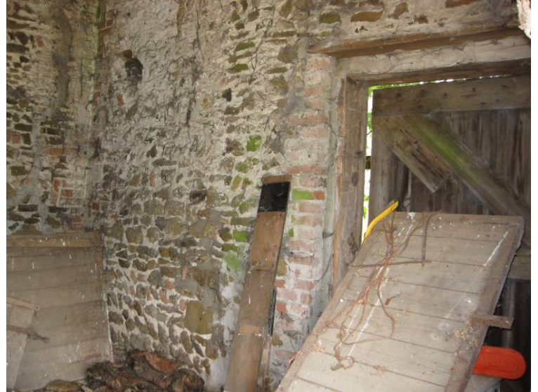
Plate 22 Interior of stable/loose box 2. Note hole in wall close to corner of room, possibly marking location of former hay rack, looking northeast
