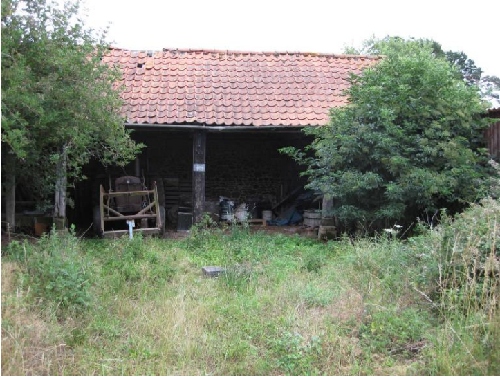
Plate 38 Cart shed frontage, looking west.
