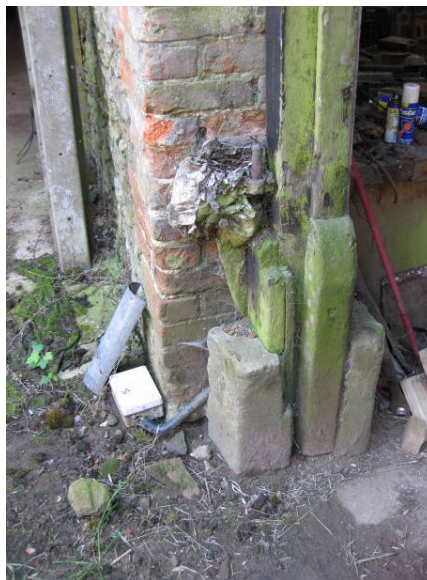
Plate 6 Detail of northern wall of main barn. Stone and wood slot at base of threshold. See also similar detailing in opposing side (Plate 5), looking east.
