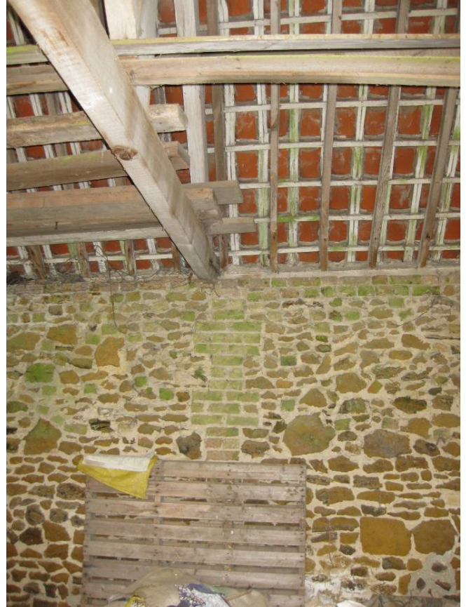
Plate 40 Detail of east wall construction in interior of cartshed, looking east.
