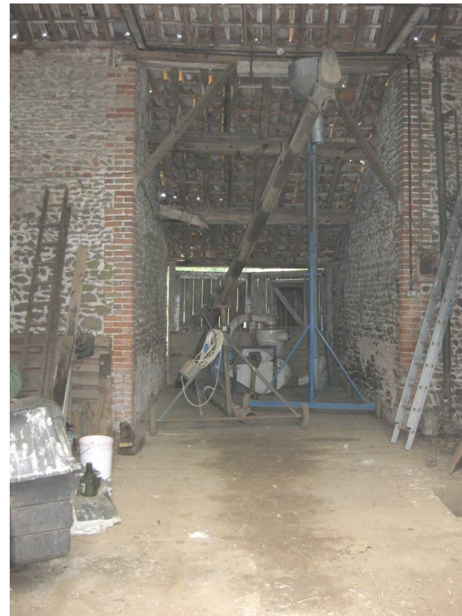
Plate 15 Interior of main barn showing view from northern doorway to barn porch, looking south.
