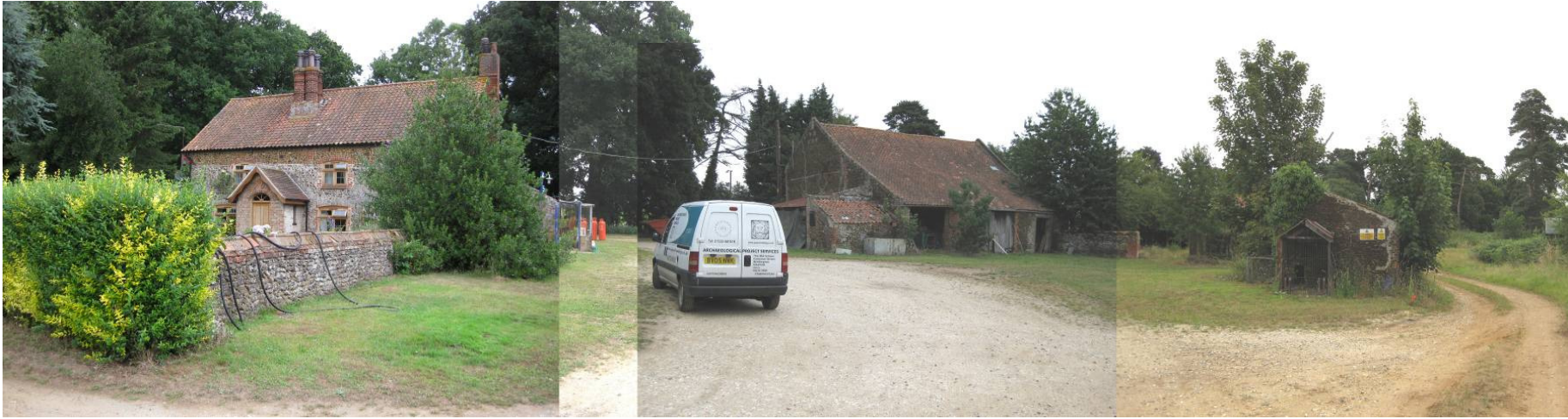
Plate 1 General view of site showing farmhouse and recorded building ranges, looking north, northeast and east.
