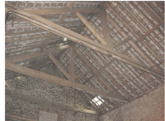
Plate 14 Interior of main barn showing detail of roof construction, looking east.
