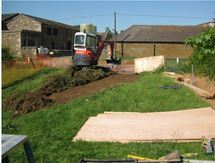
Plate 1. Topsoil stripping in progress looking south
