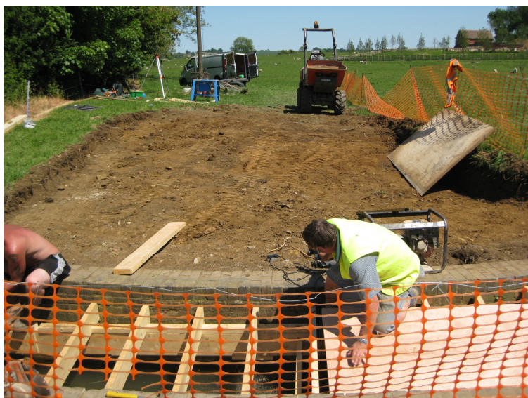
Plate 3. Completed strip for access looking northeast
