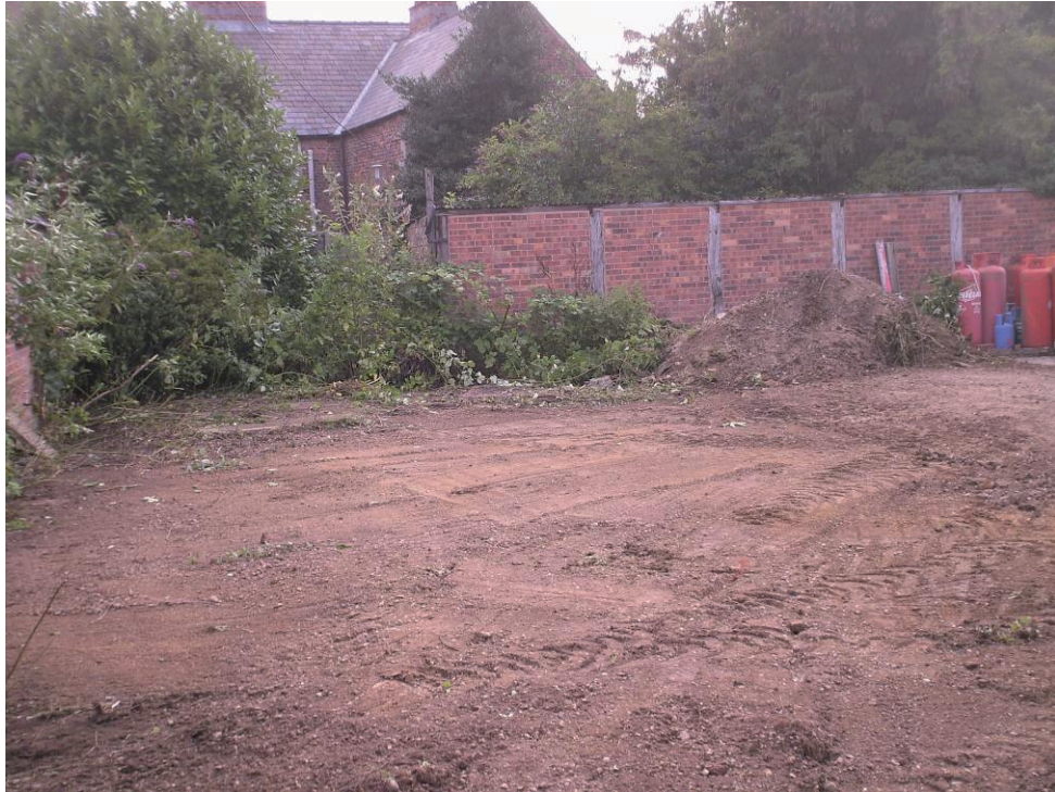
Plate 1. Pre-machining view of site looking east
