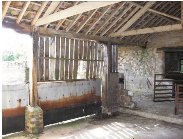
Plate 10 - Interior of open-sided shelter D showing 19 th century wooden stanchions and pillows with modern infilling, looking west
