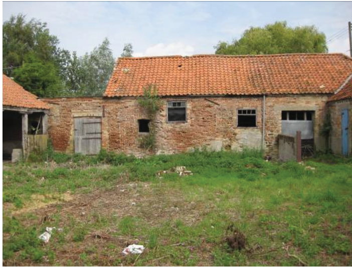
Plate 46 - Western wall of Room S viewed from Yard 4, showing various walling, features and joins of late 18 th century or earlier, 19 th century date and modern dates, looking north
