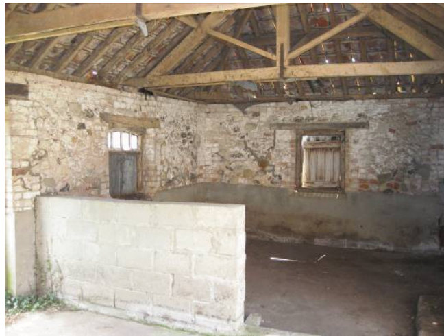
Plate 4 - Interior of Room A, showing original half-glazed window and shuttered window and modern breeze block pens, looking south
