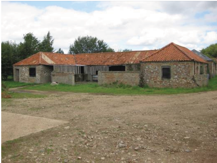
Plate 2 - View of Yard 1, Rooms E, F, D & A, looking north
