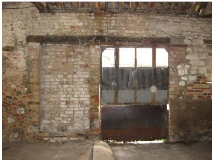
Plate 50 - Doorway in southern wall of Room S with partially modern surround, but possibly being a 19 th century doorway for a sliding door, looking south
