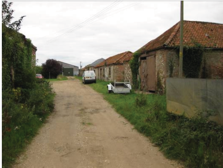
Plate 1 - General view of surveyed building range, looking southwest
