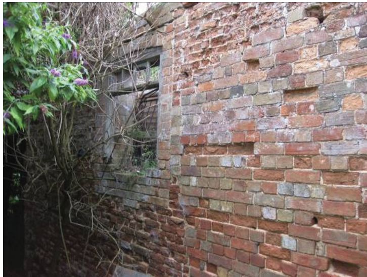
Plate 59 - Exterior of western wall of Room S showing late 18 th century or earlier brickwork with 19 th century half-glazed window, and 19 th century brickwork blocking an earlier doorway, looking east
