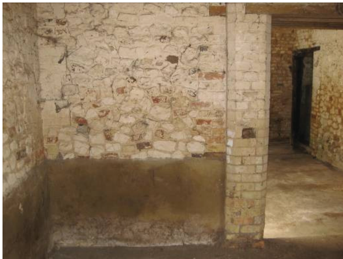
Plate 33 - Detail of notches adjacent to doorway and near corner of Room P, possibly being traces of former structures such as feed troughs or partitions, looking south
