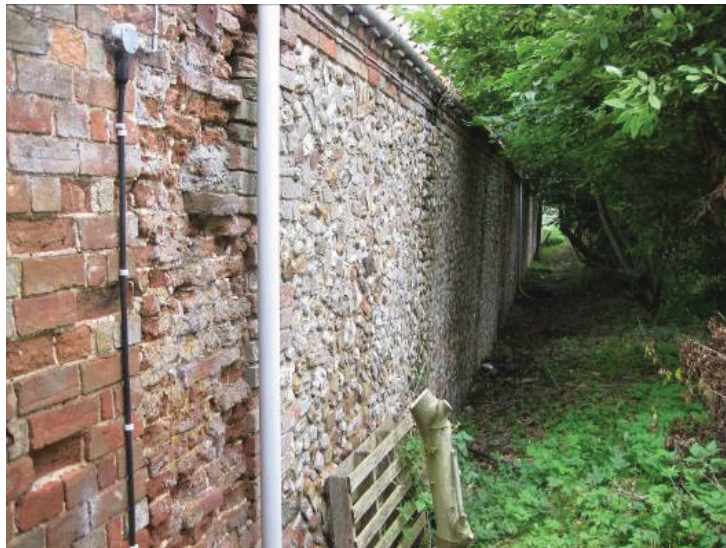
Plate 60 - Western wall of Room T, looking south
