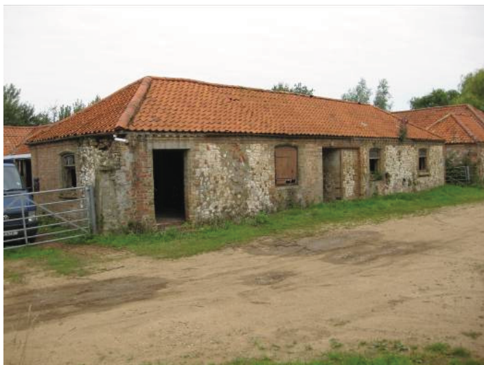
Plate 27 - Frontage of rooms N, O and P, showing 19 th century shuttered window, half-glazed windows and doorways for sliding doors, looking north
