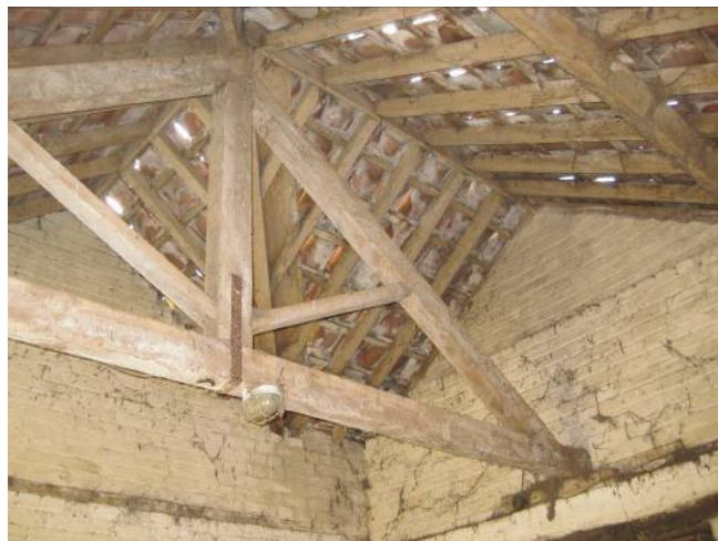
Plate 6 - Detail of roofing inside Room B, looking southwest
