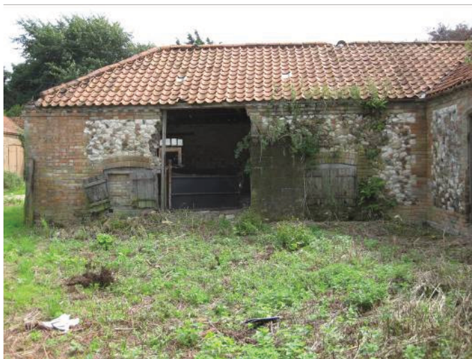
Plate 35 - Room P as viewed from Yard 4, showing 20 th century repair to walling at left and opening widened in 20 th century. Blocked low openings of 19 th century date with probable original shutters flank doorway, looking east
