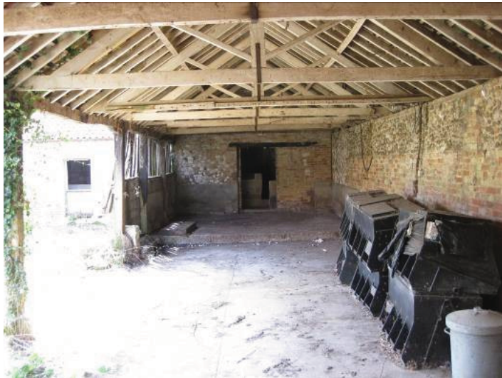
Plate 38 - Interior of open-fronted shelter T, showing doorway for sliding door at south, looking south
