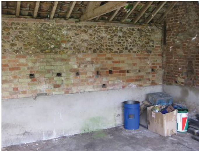
Plate 40 - Interior of open-fronted shelter T, showing series of holes in western wall possibly relating to former hay rack, looking north
