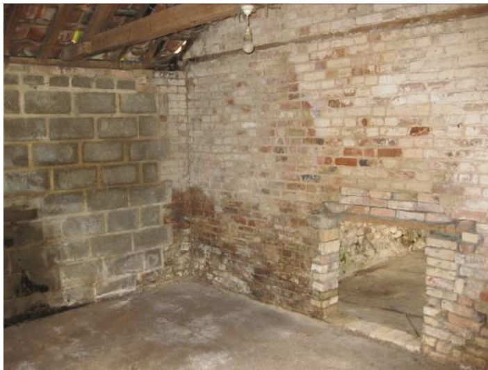
Plate 29 - Interior of Room N showing 19 th century walling at right with probable modern low opening, and modern breeze block western wall, looking north
