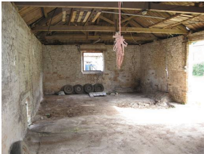
Plate 21 - Interior of Room J, looking northeast
