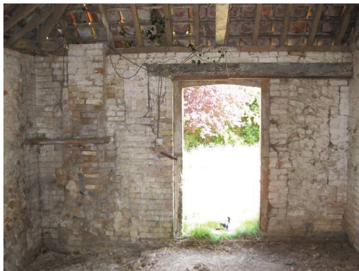
Plate 61 – Former sliding door and adjacent possible chimney, Room B
