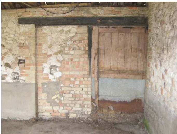
Plate 18 - Detail of 19 th century sliding door in north wall of open-sided shelter I with some modern repairs to brickwork, looking north
