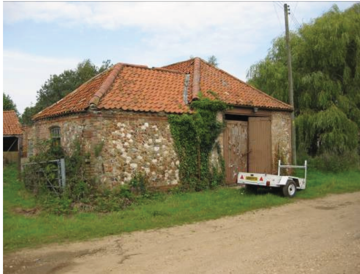
Plate 34 - Frontage of Rooms R and S showing large modern doors to Room S, looking north
