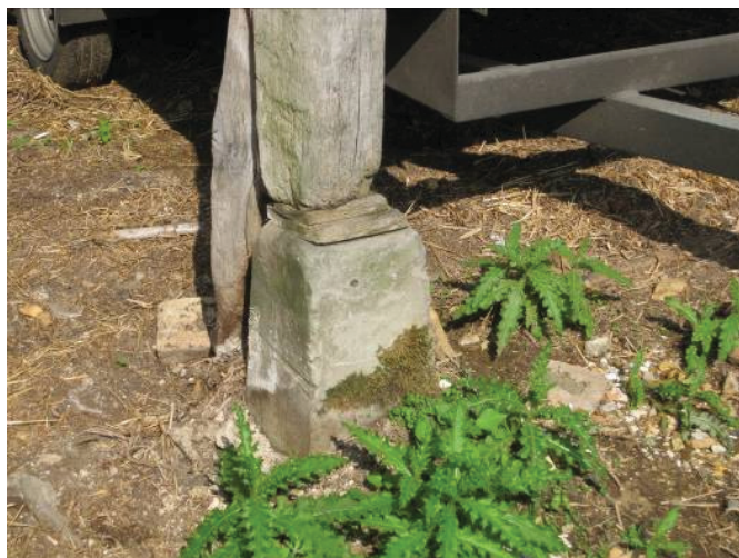
Plate 24 - Detail of 19 th century stone stanchion base and timber stanchion of Shelter K, looking northwest
