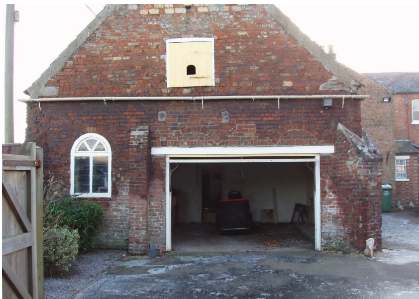
Plate 3 North elevation, showing blocked window arches, looking southwest
