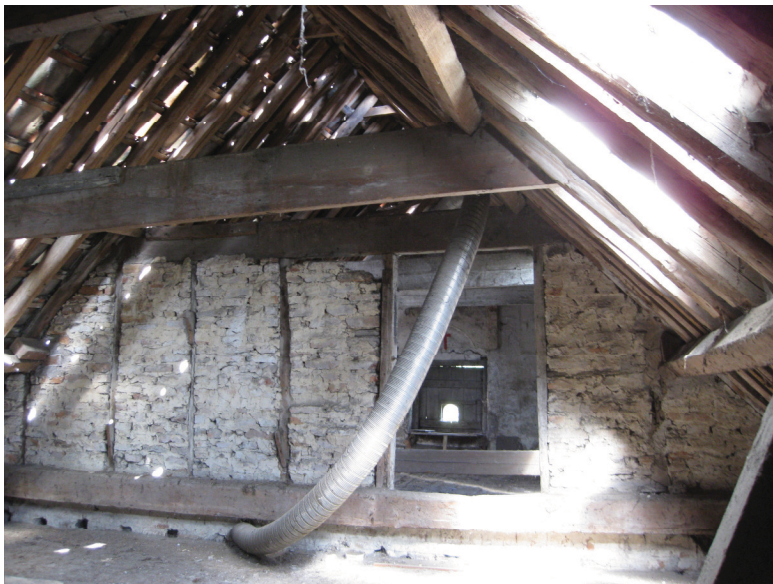
Plate 17 Upper storey, southern surveyed room, looking northeast
