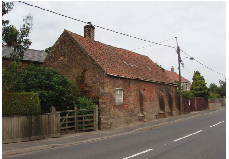
Plate 8 South and east elevations, looking north
