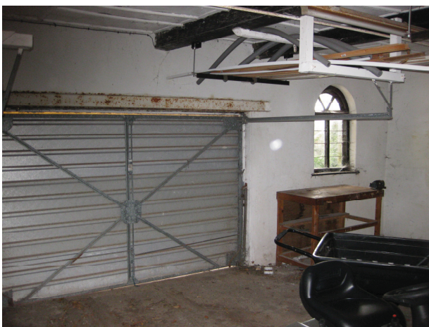
Plate 14 Ground floor, north room, showing window and garage door, looking east
