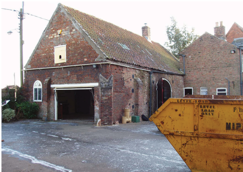
Plate 2 North and west elevations of recorded building, looking south
