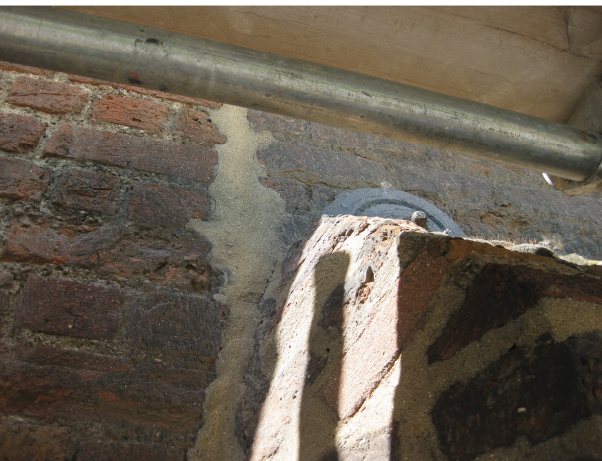
Plate 6 Detail of straight joint adjacent to buttress, looking west
