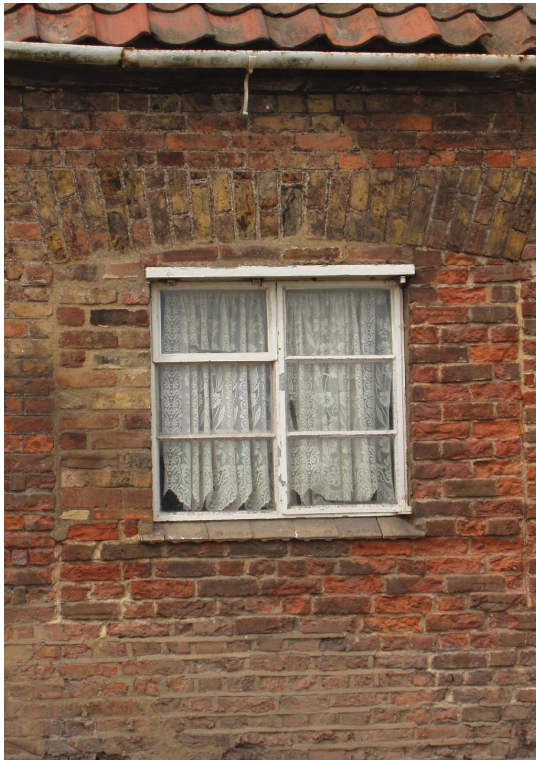
Plate 7 Detail of inserted and blocked window, eastern elevation, looking west
