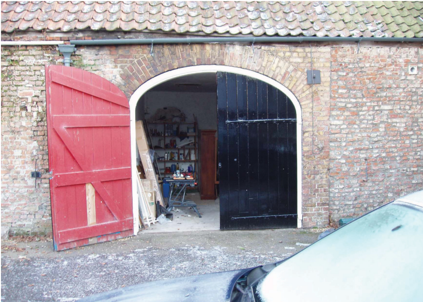
Plate 4 Western elevation, inserted doorway, looking southeast
