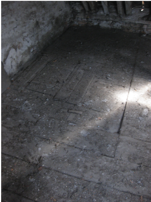
Plate 20 Upper storey, northern room, trapdoor and patched floor in northeastern part of room, looking east
