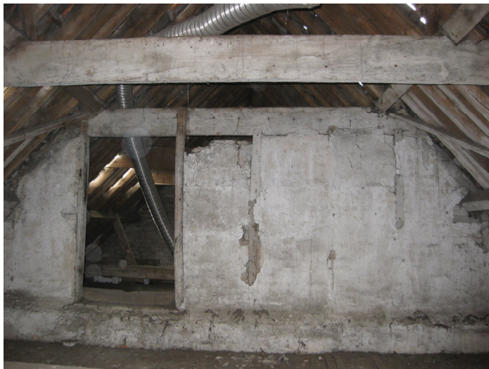
Plate 19 Upper storey, northern room, showing partition wall between rooms, looking south
