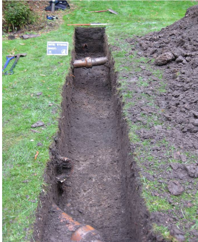
Plate 2 – General view of western footing, looking north
