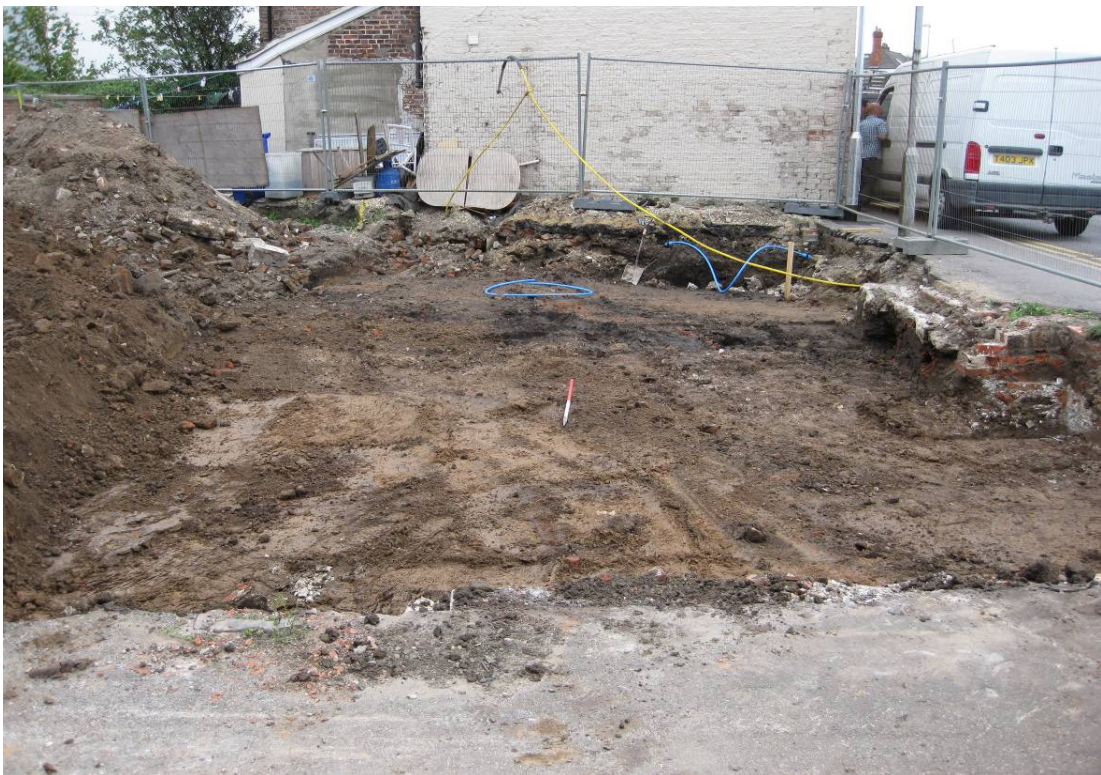
Plate 2 – Area of ground reduction looking south-east
