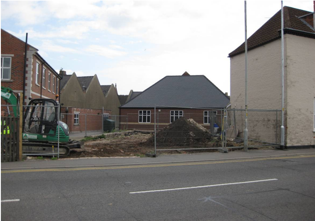
Plate 1 – General view of site looking north-east
