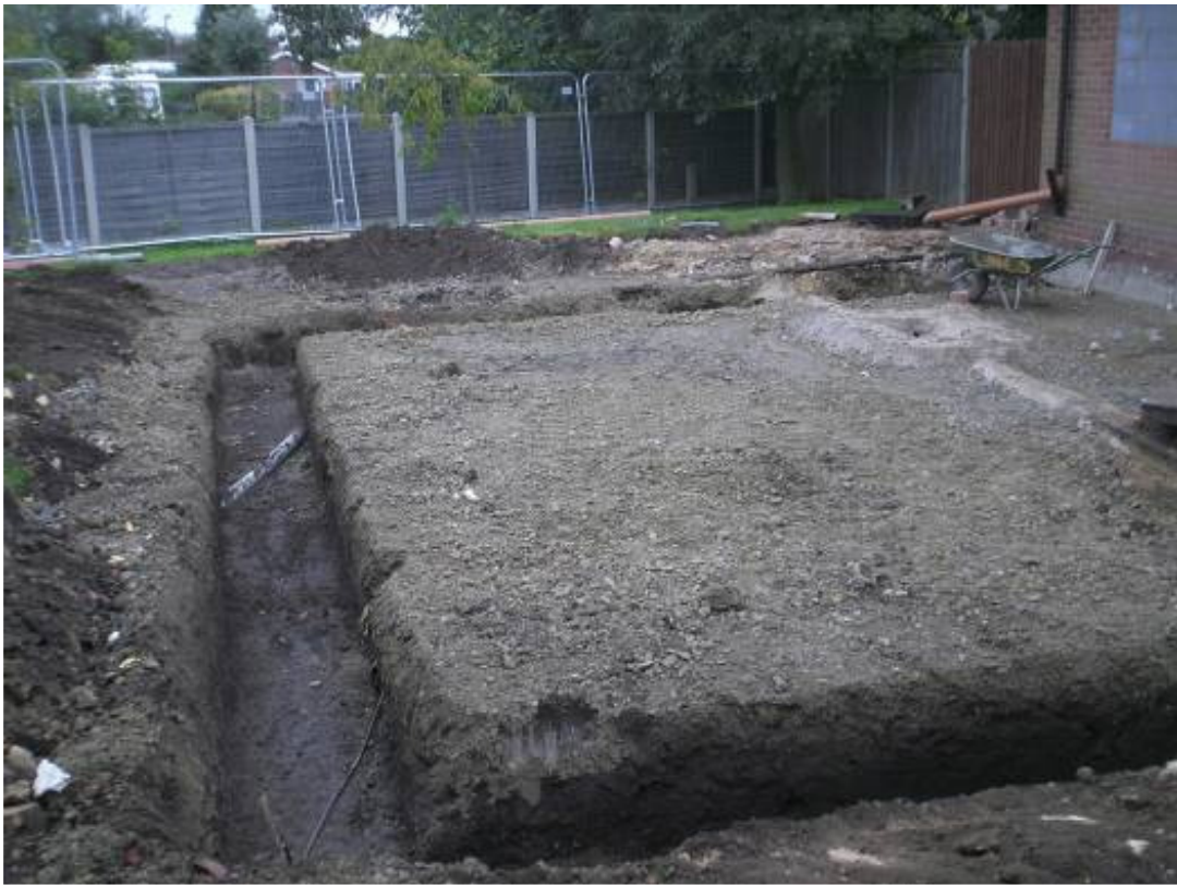
Plate 3: Area one footing trenches
