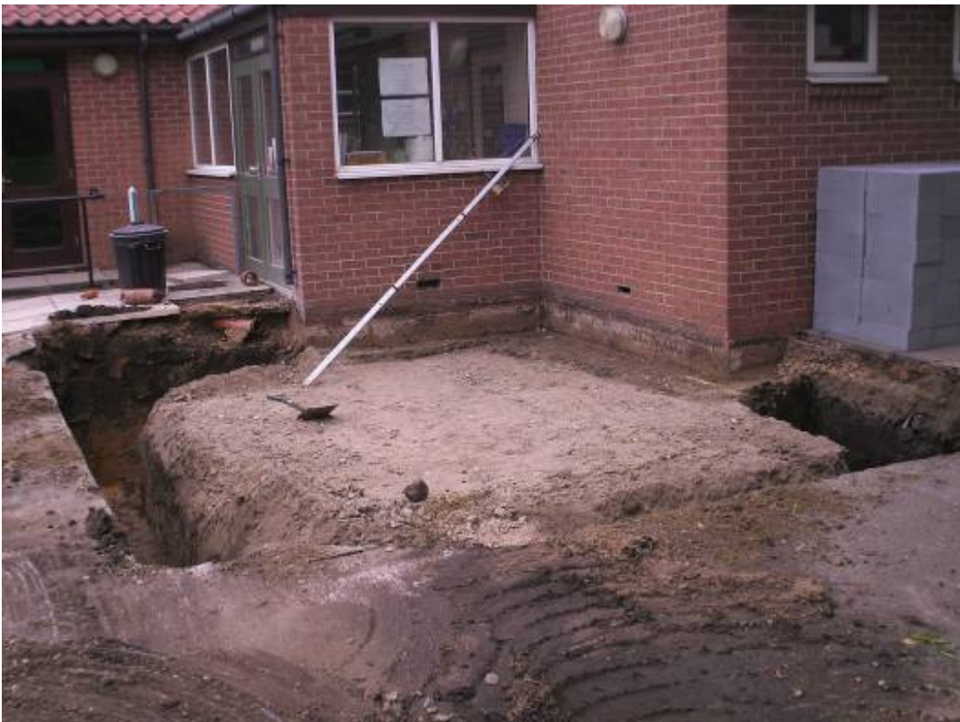
Plate 6: Area two footing trenches
