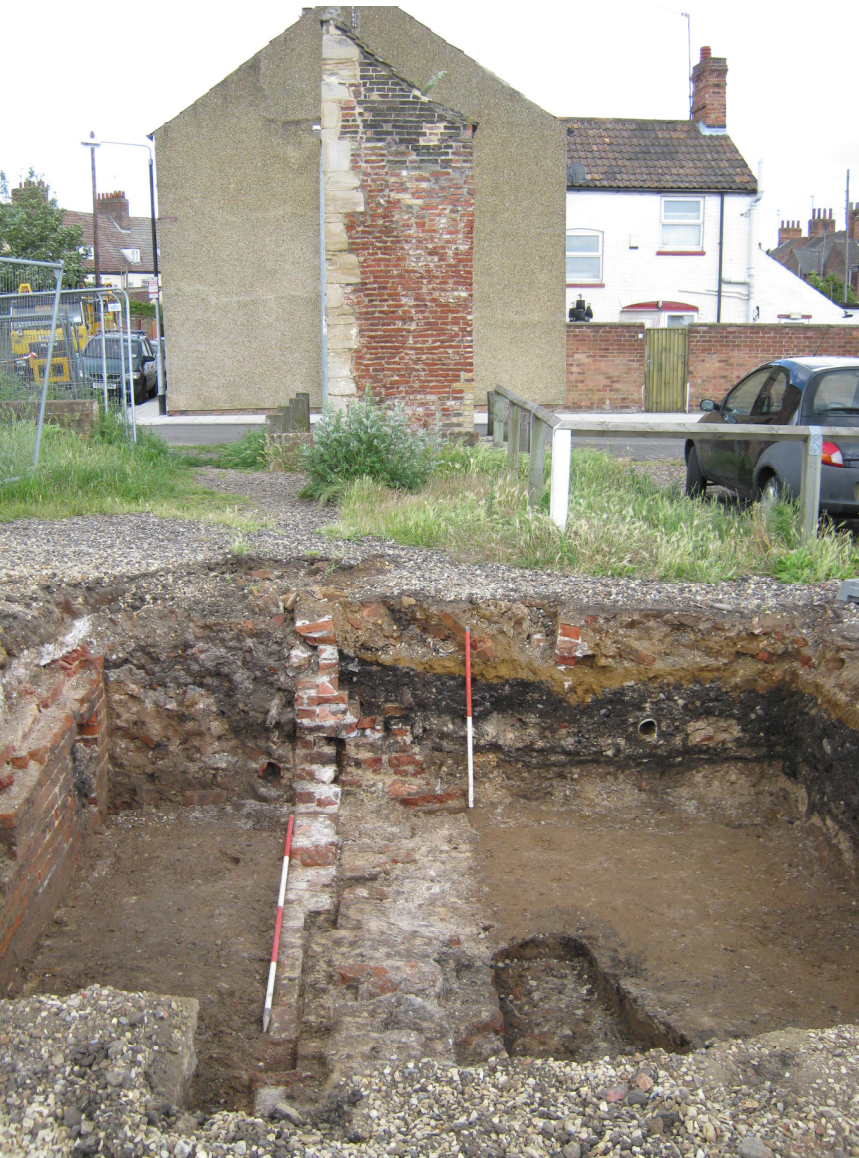
Plate 20 – Trench 7: Section 42 with the Carmelite Arch in the background, looking east
