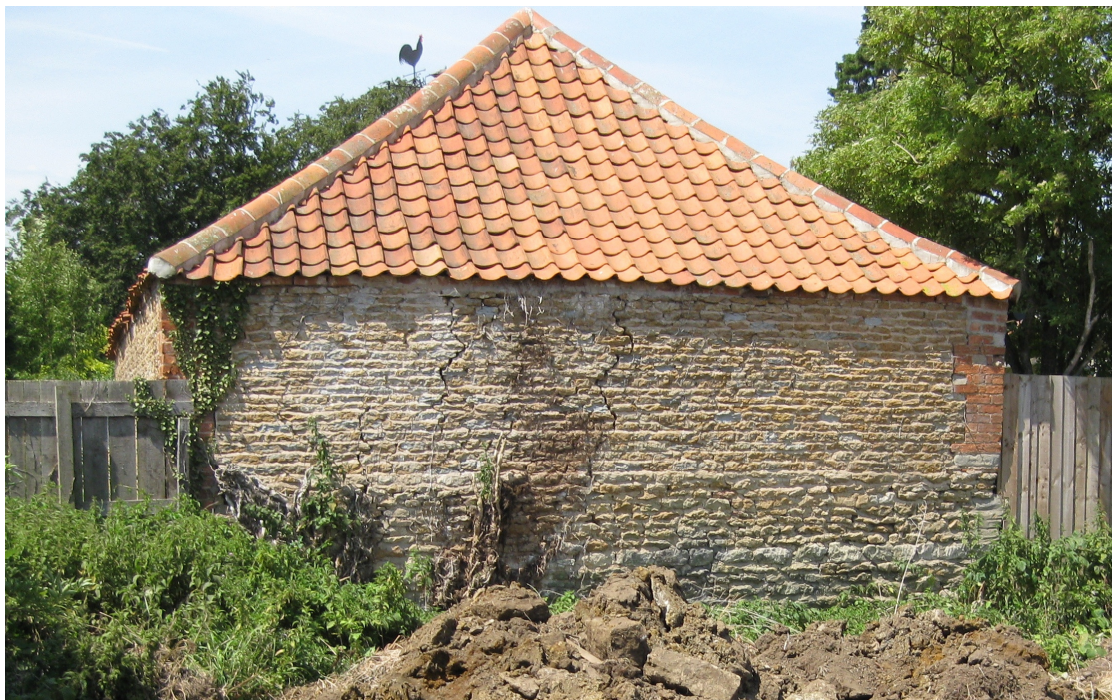
Plate 4. Building at southwest of site, looking west
