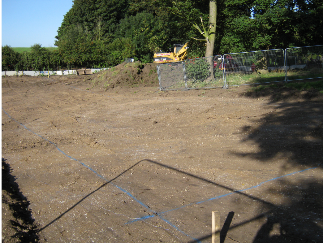
Plate 1. General view of marked out site following topsoil stripping looking west
