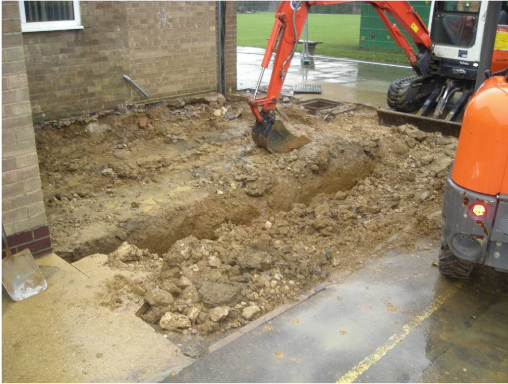
Plate 1 – Excavation of Trench 1, looking northeast
