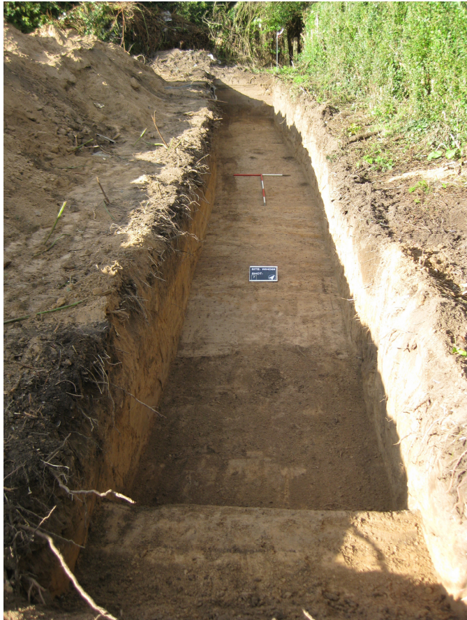
Plate 3. Plan shot of Trench 1 looking northwest with backfilled sondage in foreground
