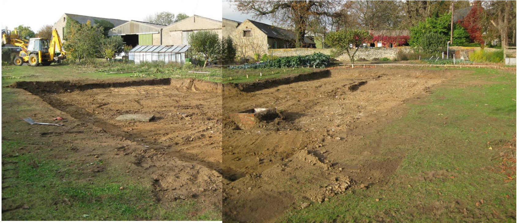
Plate 1 General view of stripped bungalow area, looking northwest
