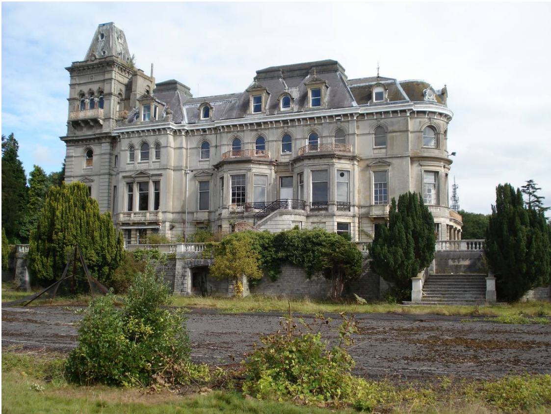
Plate 4 – View of the west front of the house prior to the present works, showing the terrace wall and late 20 th century tennis courts which were built within the area of the formal gardens
