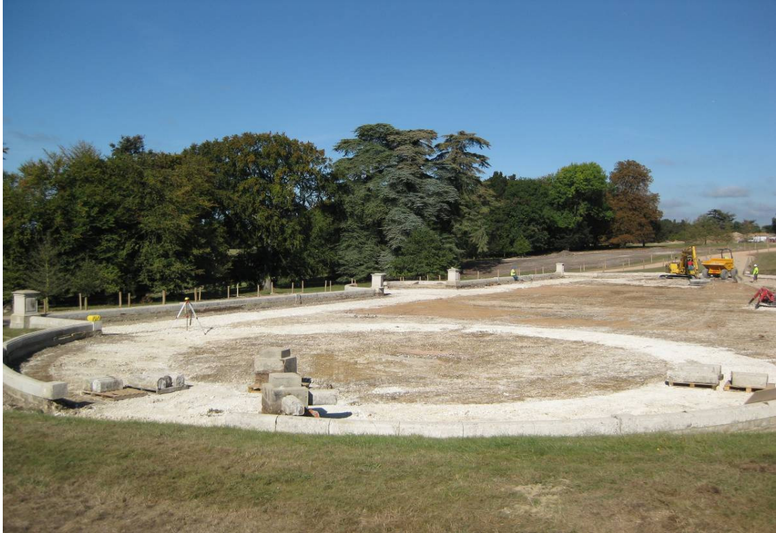
Plate 7 – Southern end of formal gardens after ground reduction
