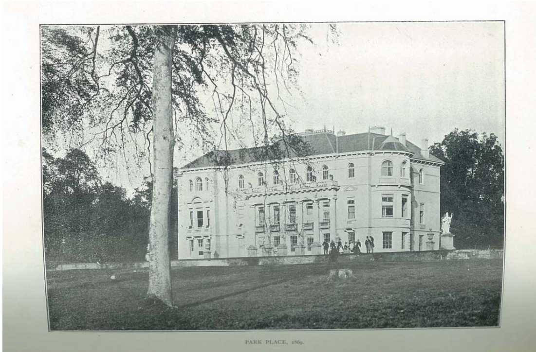
Plate 1 - View of the west front of the house from 1869 showing the previous terrace wall prior to the construction of the formal gardens
