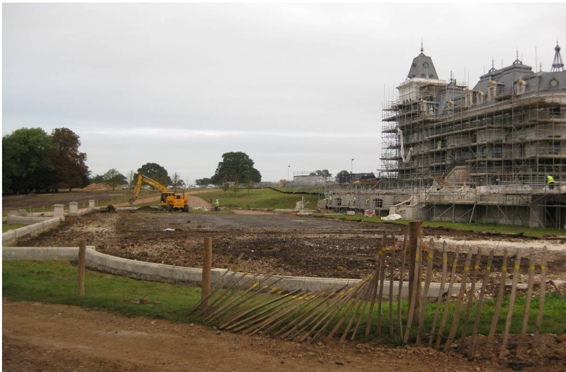
Plate 6 – Removal of topsoil and tennis courts in progress
