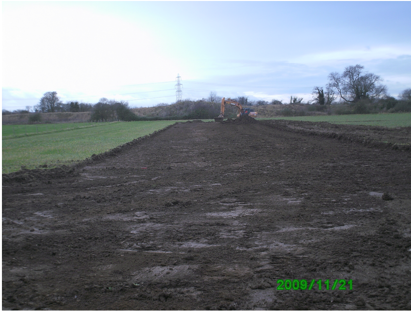
Plate 3. Machining area of poultry units looking west
