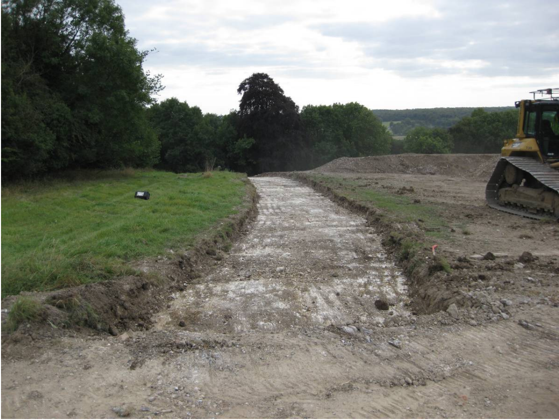
Plate 15 – Northern end of new road, looking south
