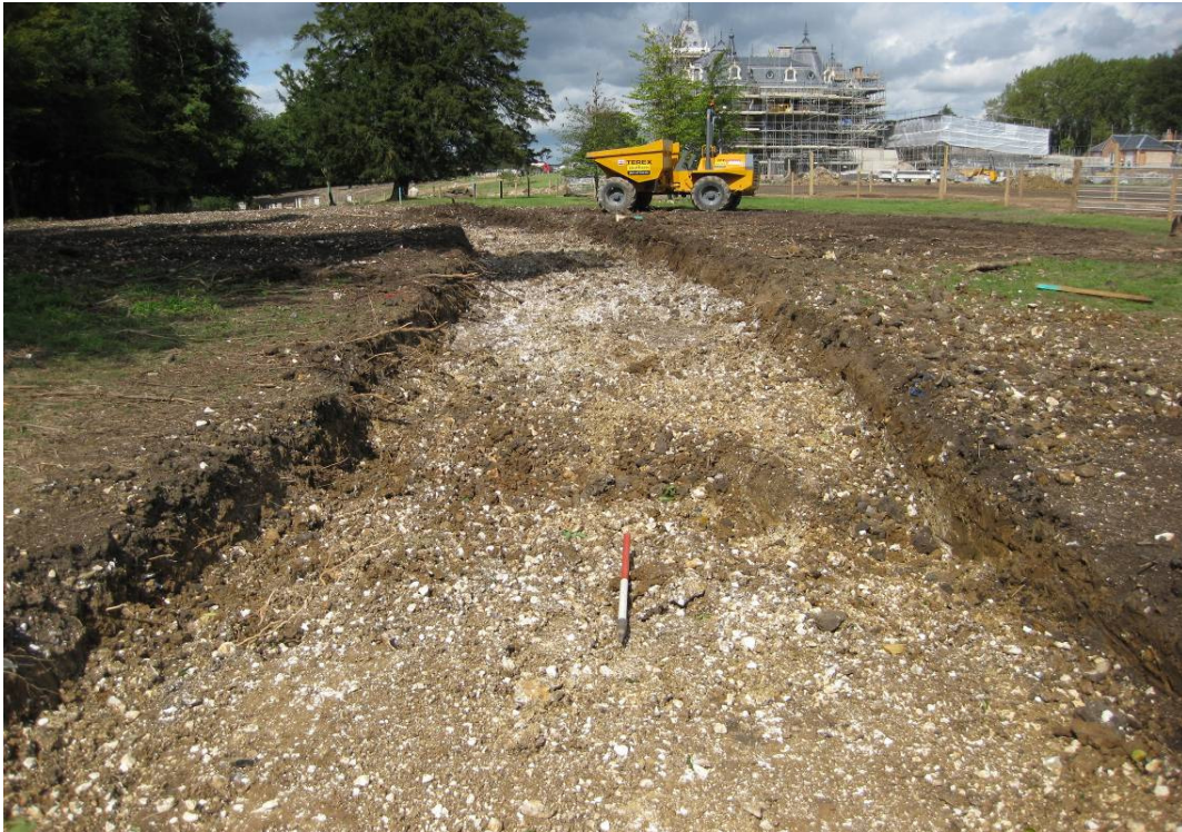
Plate 1 – New road, looking north
