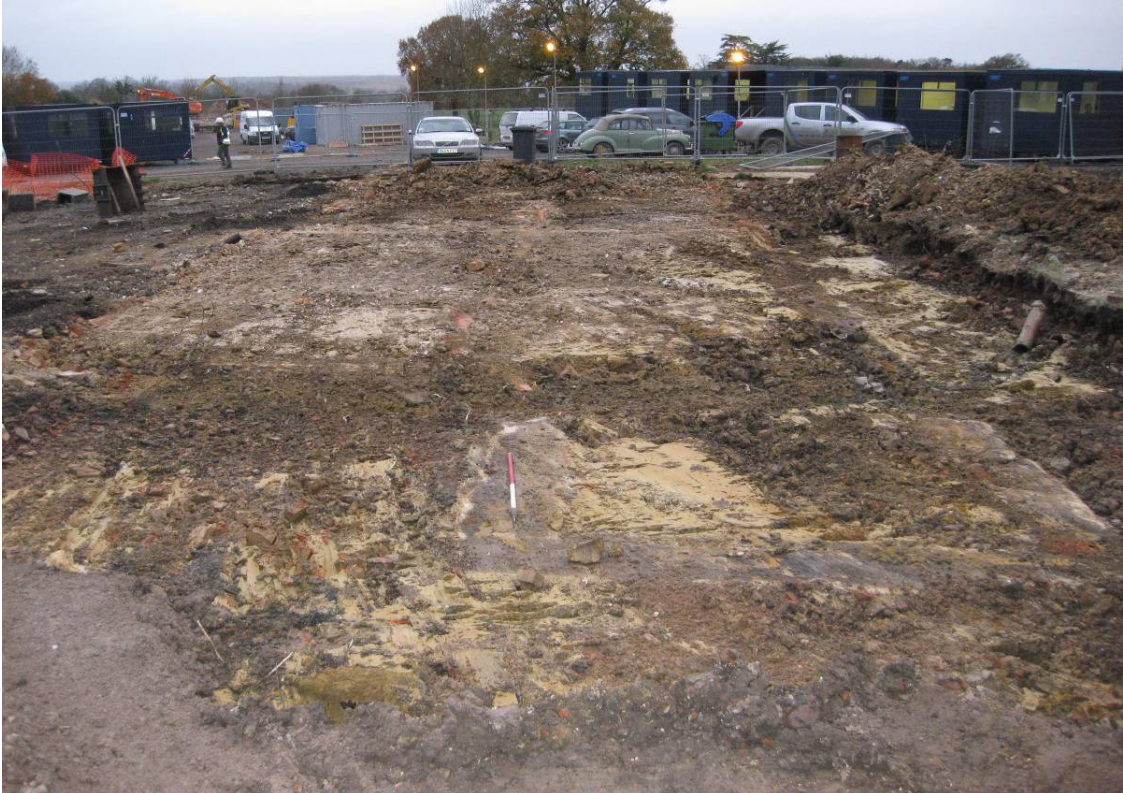
Plate 2 – Area underneath concrete slab looking north-west
