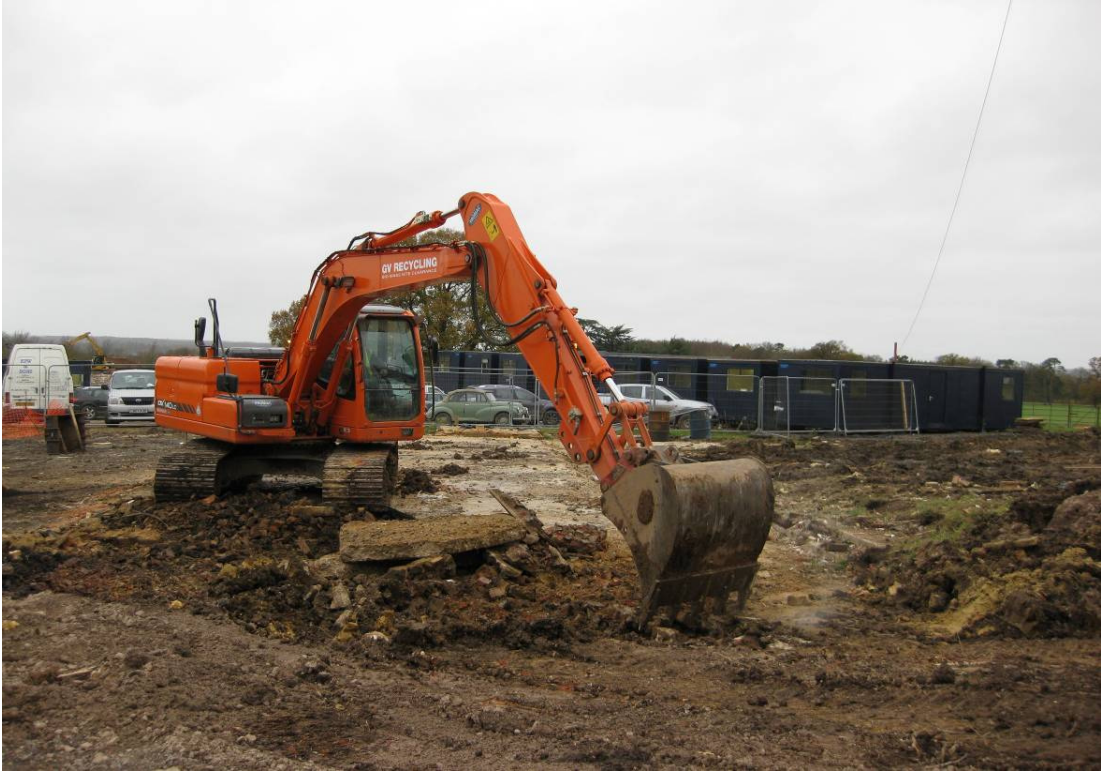
Plate 1 – Removal of concrete slab
