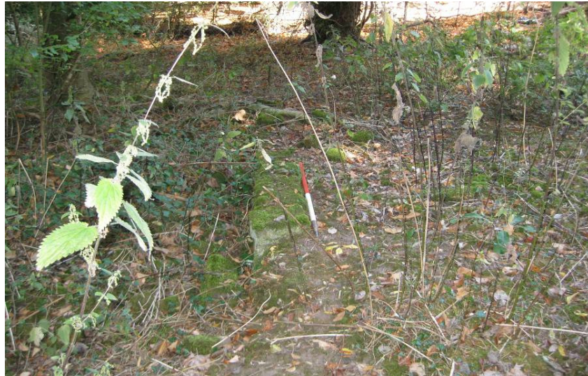
Plate 3 – Foundations of the Chinese Cottage
