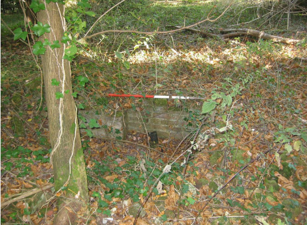
Plate 1 – Foundations of the Chinese Cottage
