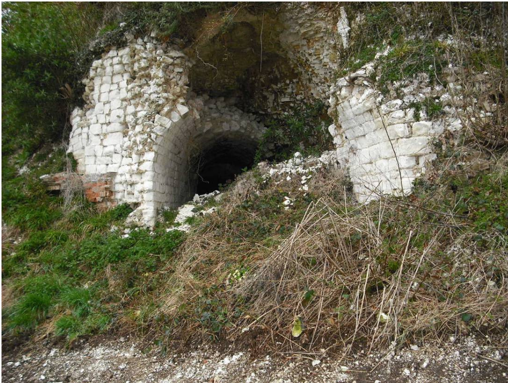
Plate 7 – Westernmost arch (entrance to tunnel) of Grecian Grotto prior to current work
