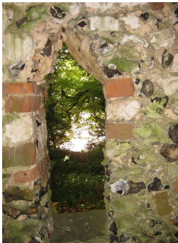
Plate 25 – View through the northern window of the Flint Gazebo
