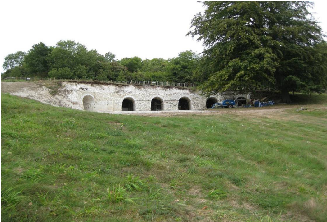
Plate 13 – View of the Grecian Grotto taken during the current program of reconstruction and consolidation
