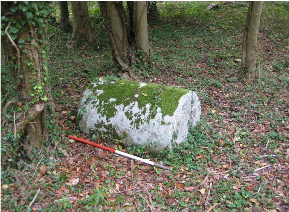
Plate 39 – Missing section of stone column to the west of the house
