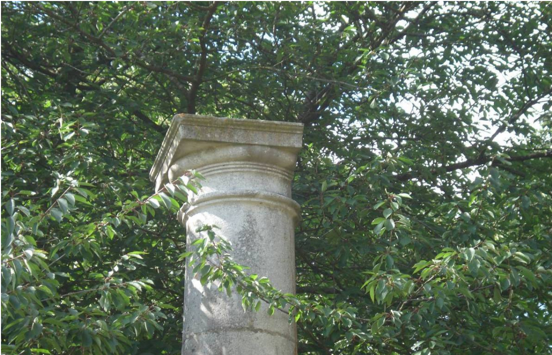
Plate 35 – Stone column located to the east of the house, showing the squared off top where it was once attached to the west front of the house
