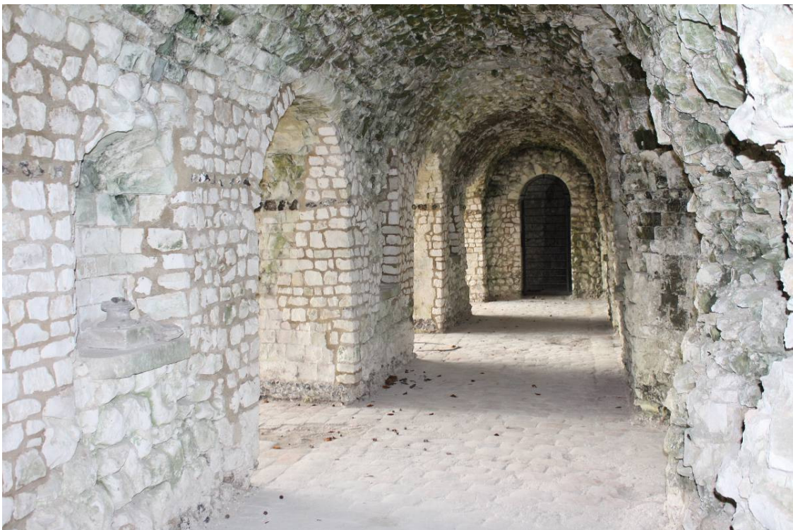
Plate 9 – Barrel vaulted space within the Grecian Grotto; note the small niche for statuary
