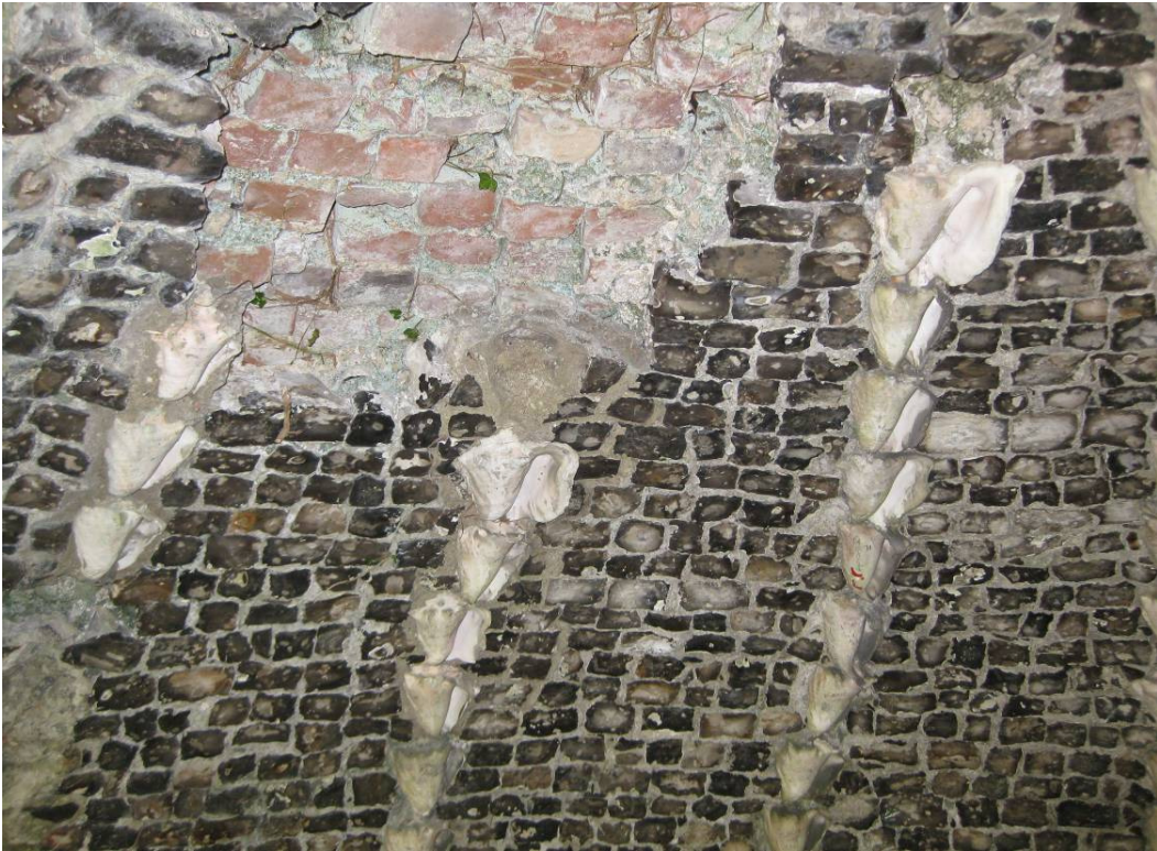
Plate 18 – View of the square knapped flints with ribs of inset conches overlying the brickwork of the Flint and Shell Alcove/Grotto
