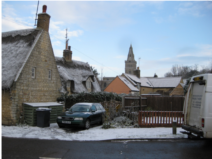
Plate 1 – View looking northwest of the development area
