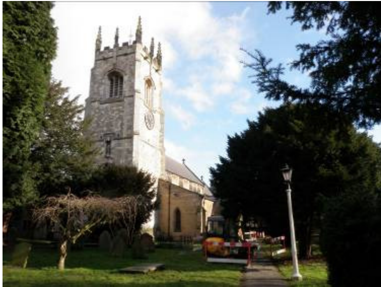
Plate 1 – St Andrew's church showing works in progress, looking east
