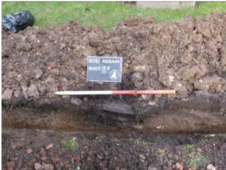
Plate 5 – Section 5 showing brick burial vault (005), looking north
