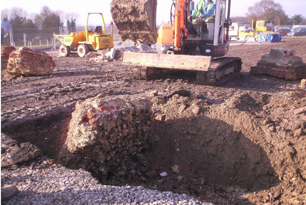
Plate 5 – Removal of obelisk foundations in Trench 2
