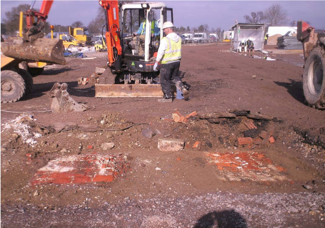
Plate 2 – Obelisk foundations in Trench 1 prior to excavation
