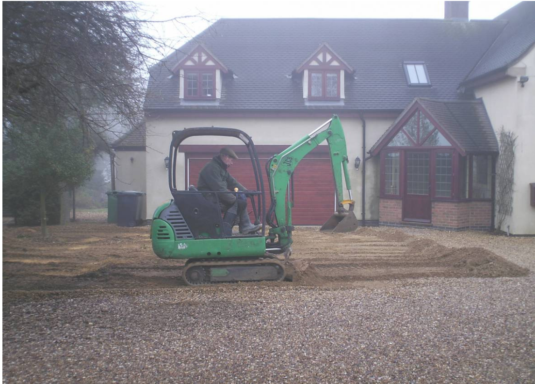
Plate 4 – Area 2 prior to excavation
