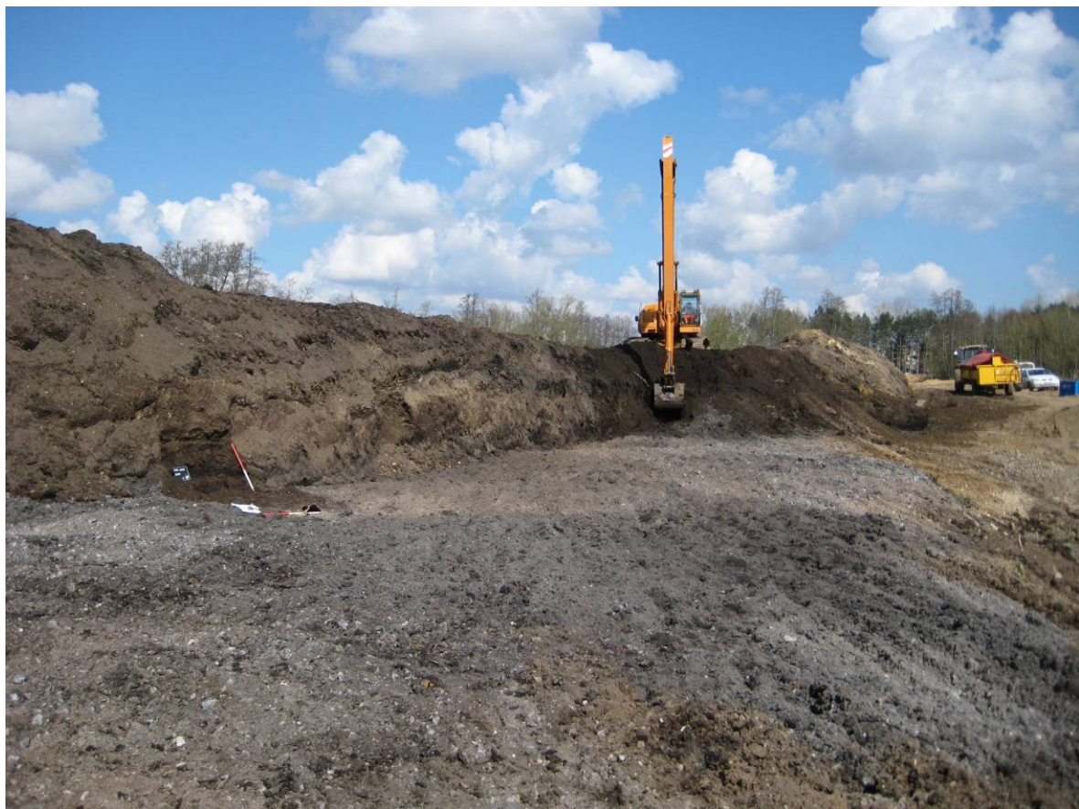
Plate 2 Peat stripping in progress
