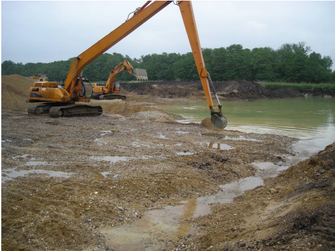
Figure 3 Gravel extraction in progress showing waterlogged conditions
