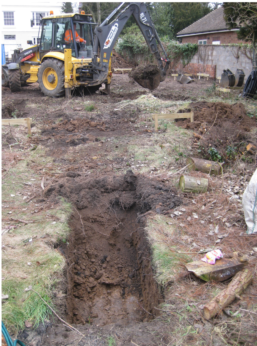
Plate 2. Machining shot with soakaway in foreground, looking northwest
