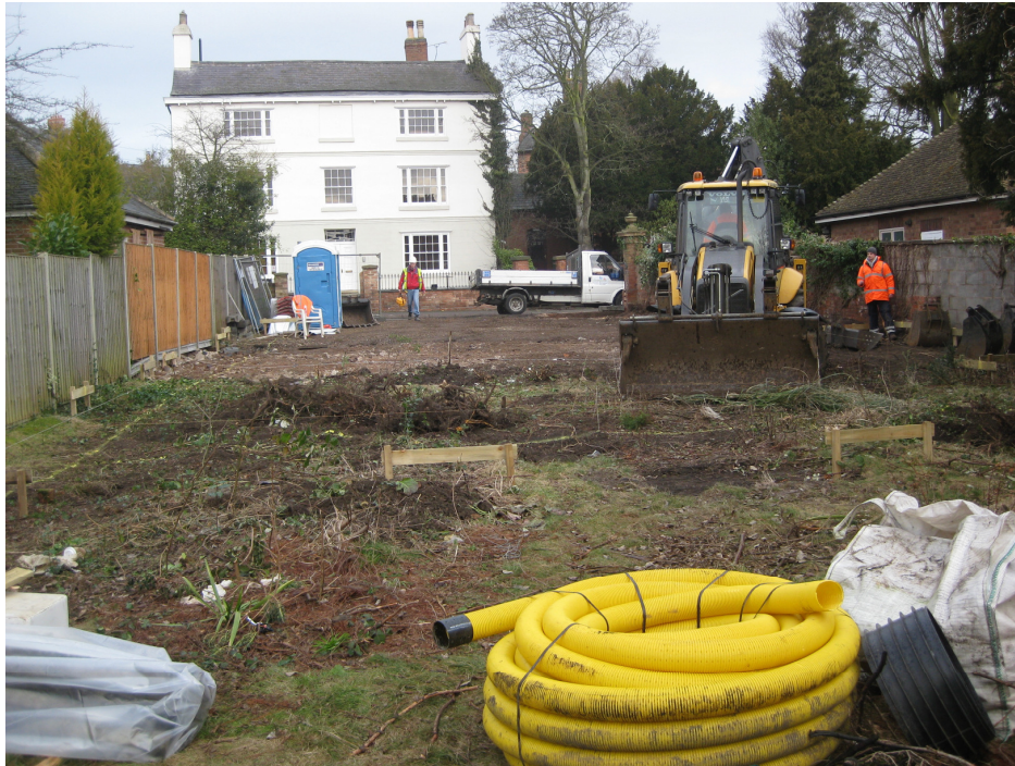
Plate 1. Pre-excavation view of site looking northwest
