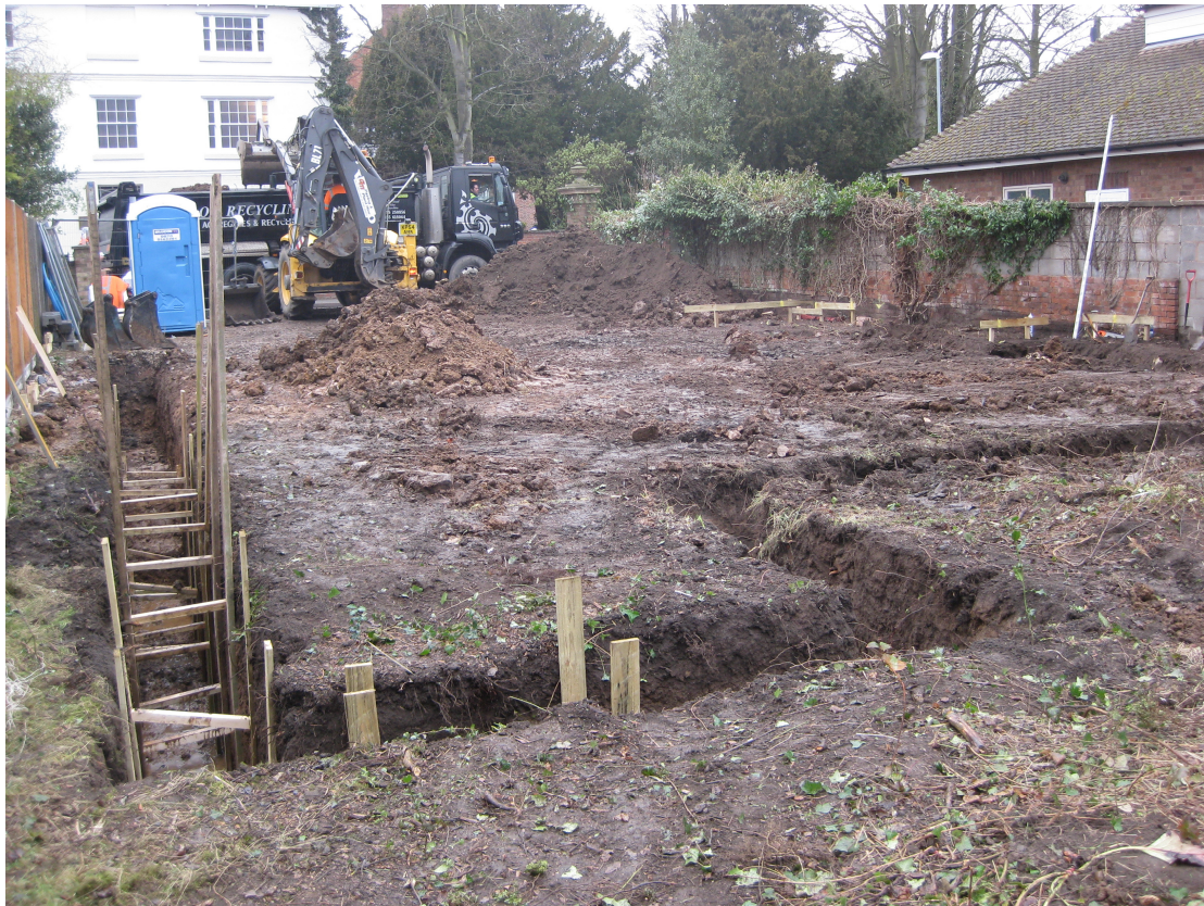
Plate 7. General view of footings looking northwest
