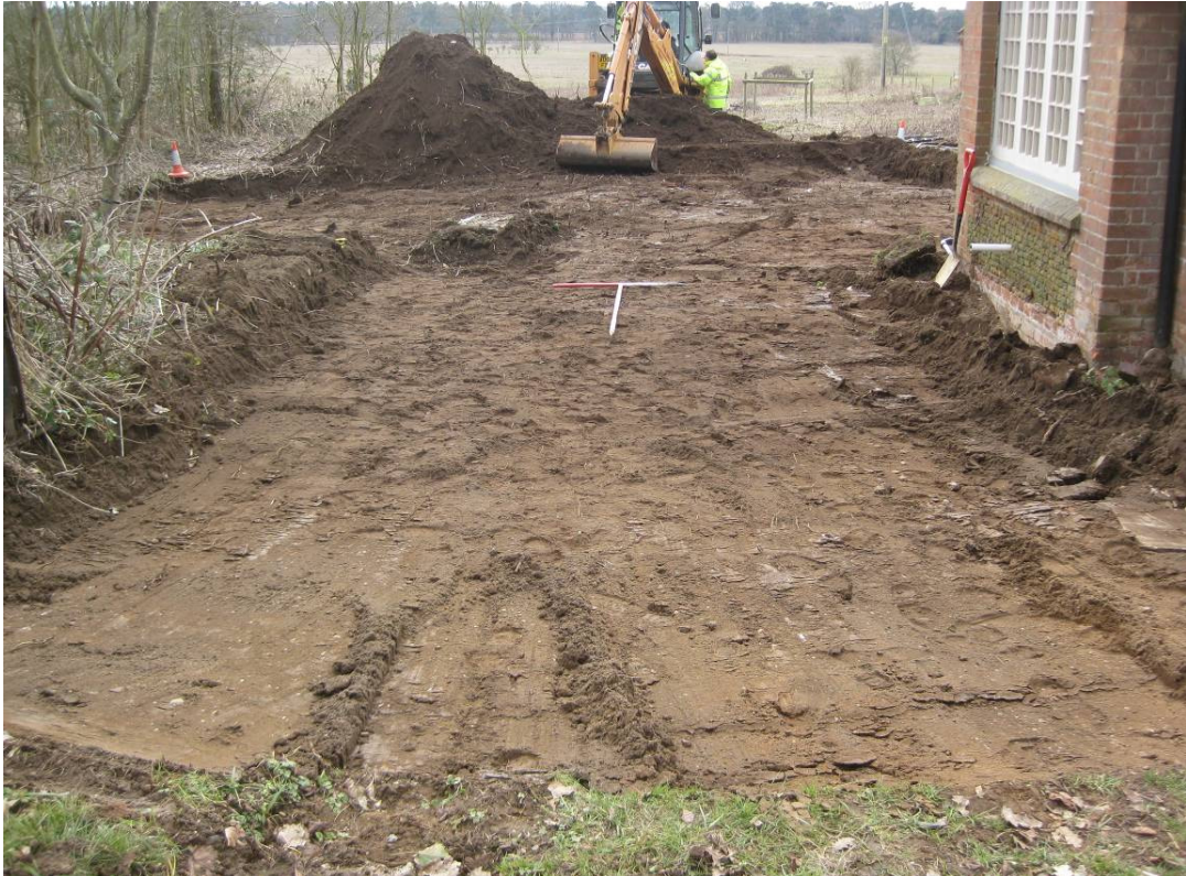
Plate 2 – General view of excavated area looking south
