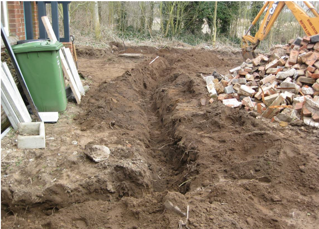
Plate 4 – View of pipe trench, looking east
