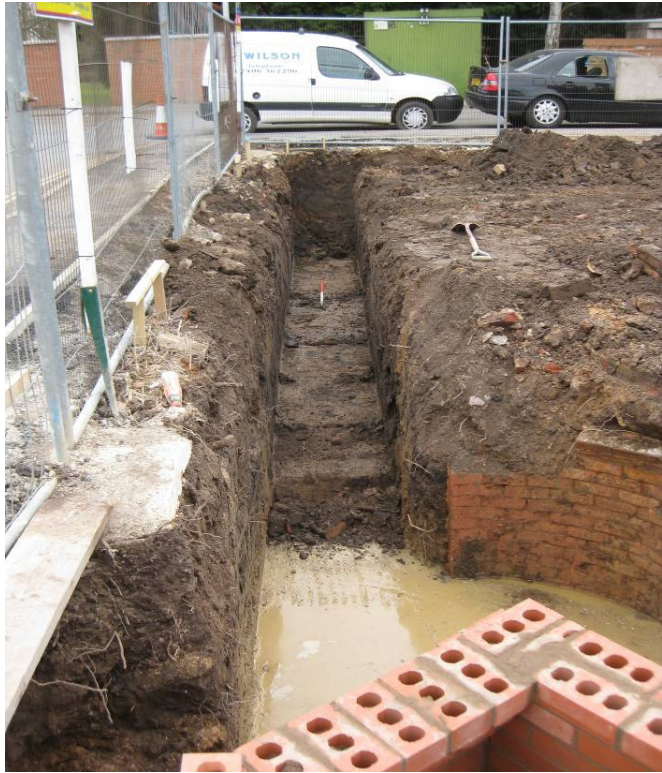
Plate 3 – View of southernmost footing looking west
