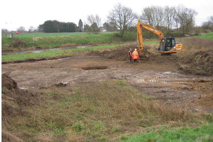
Plate 4 – Pond 2 during excavation, looking southeast
