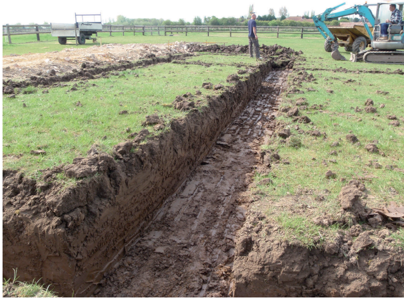
Plate 1. Machining of house footings in progress looking south
